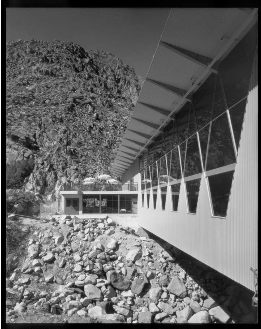
Figure 3. Southwest elevation, looking north, 1964.
