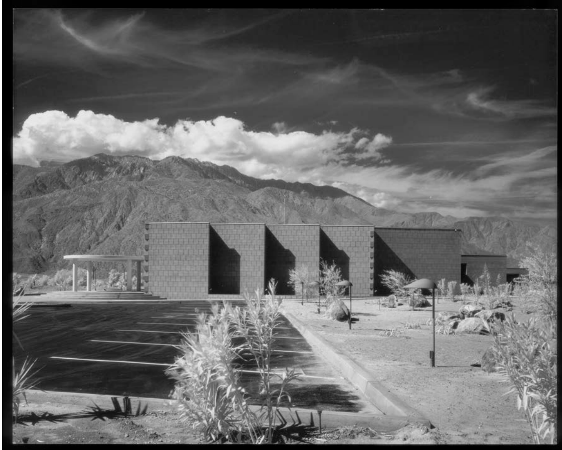
Figure 6. East elevation, looking west, 1958.
