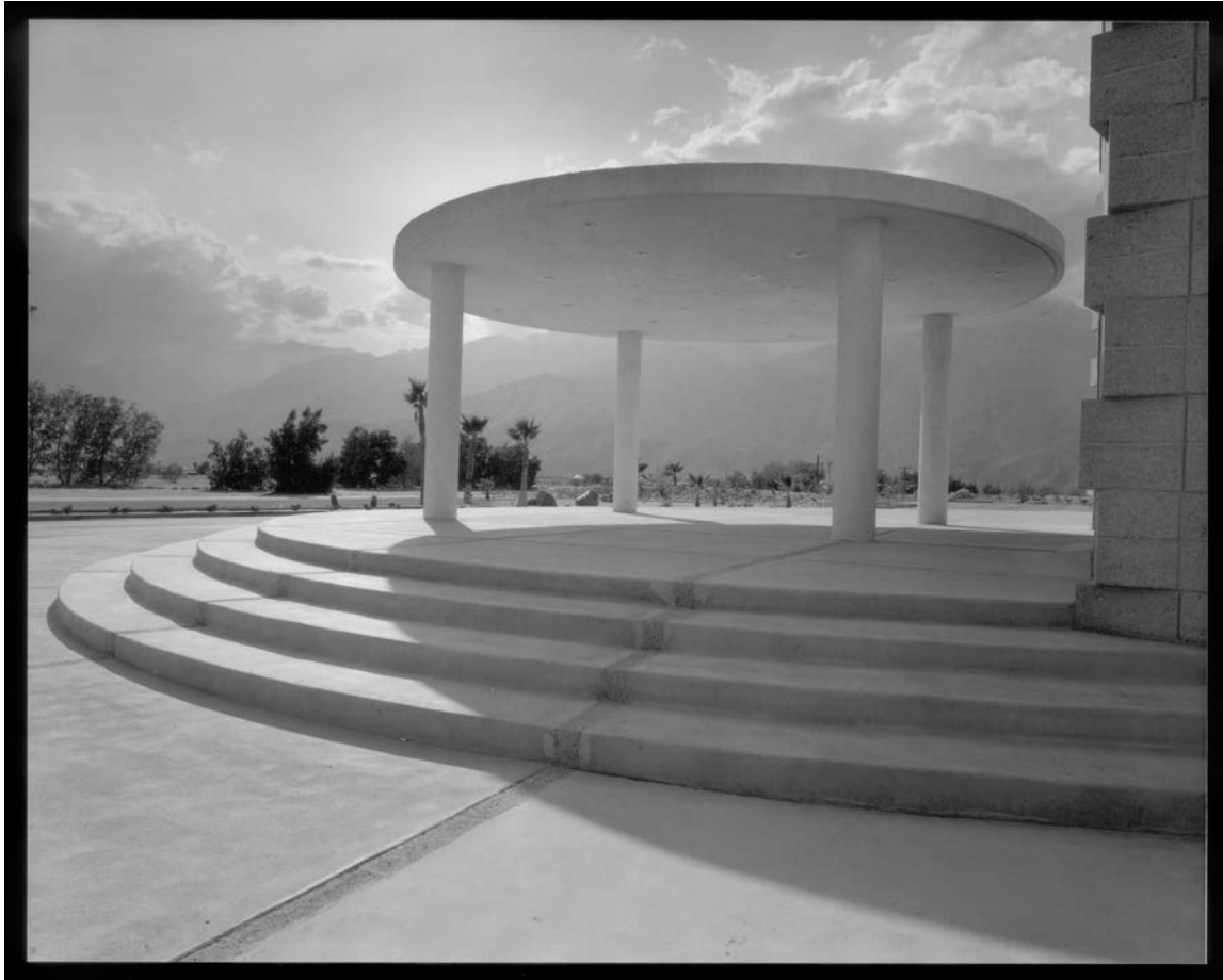
Figure 8. Detail, council chambers entrance, looking southwest, 1958.
