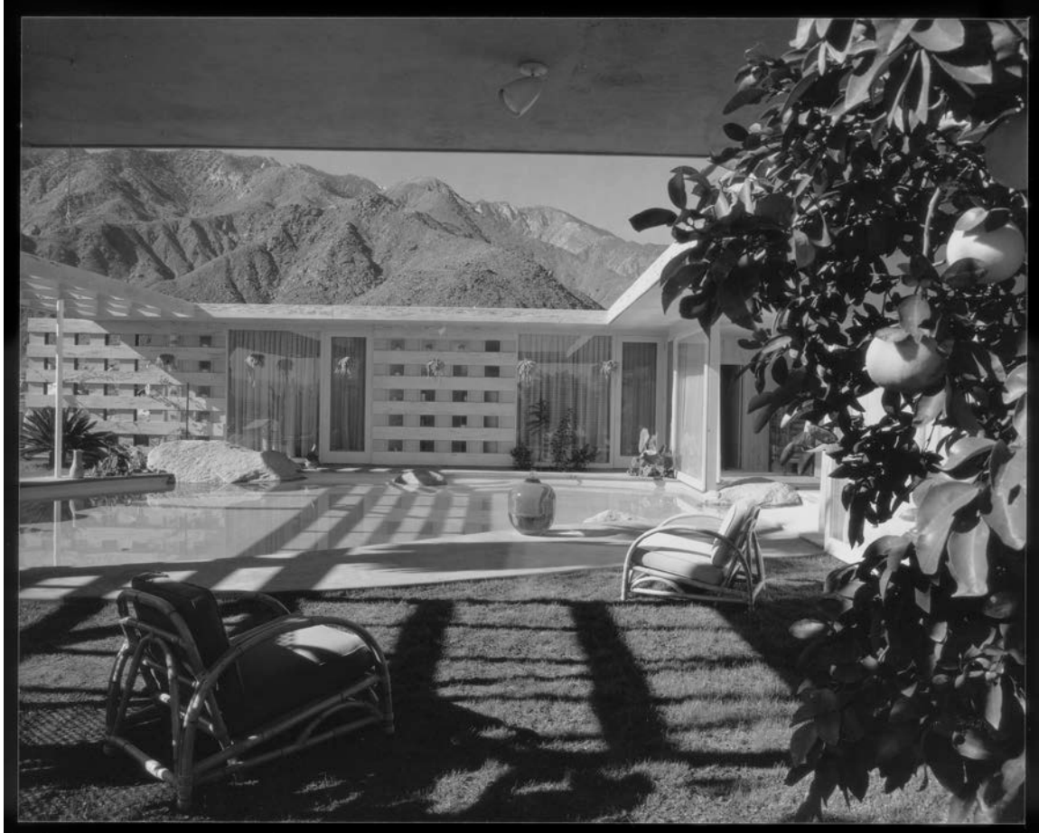
Figure 5. East elevation, looking west, 1947.
