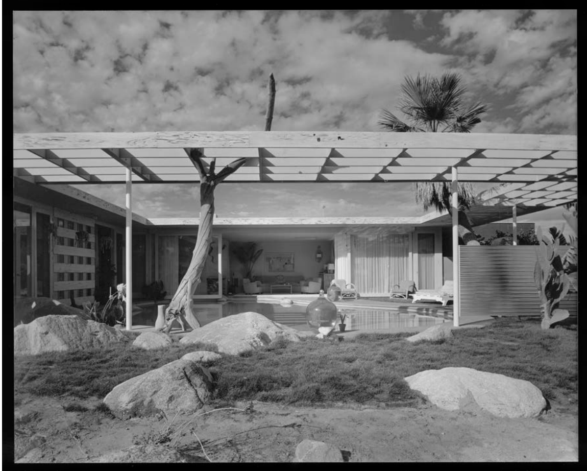
Figure 6. South elevation, looking north, 1947.
