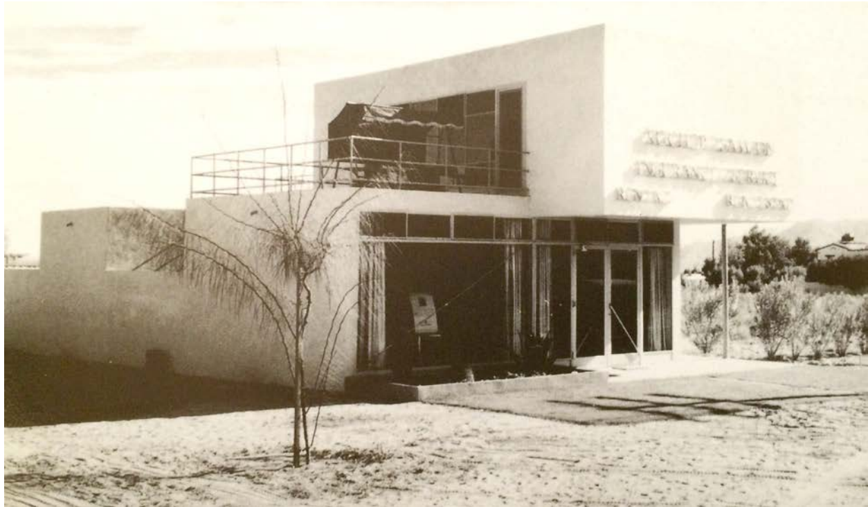
Figure 3. North and west elevations, looking southeast, circa 1935. Photo by Stephan Willard. Courtesy Palm Springs Historical Society.
