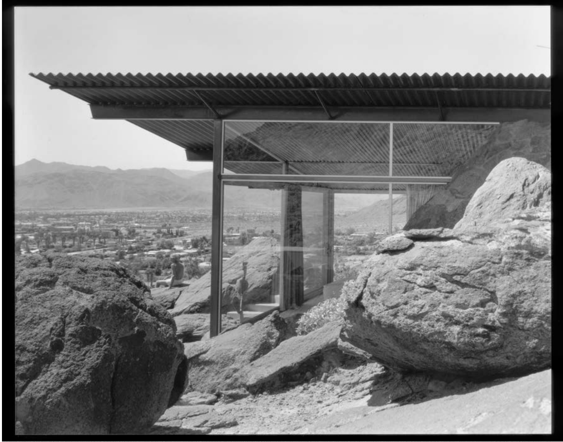
Figure 4. North elevation, looking south, 1965.
