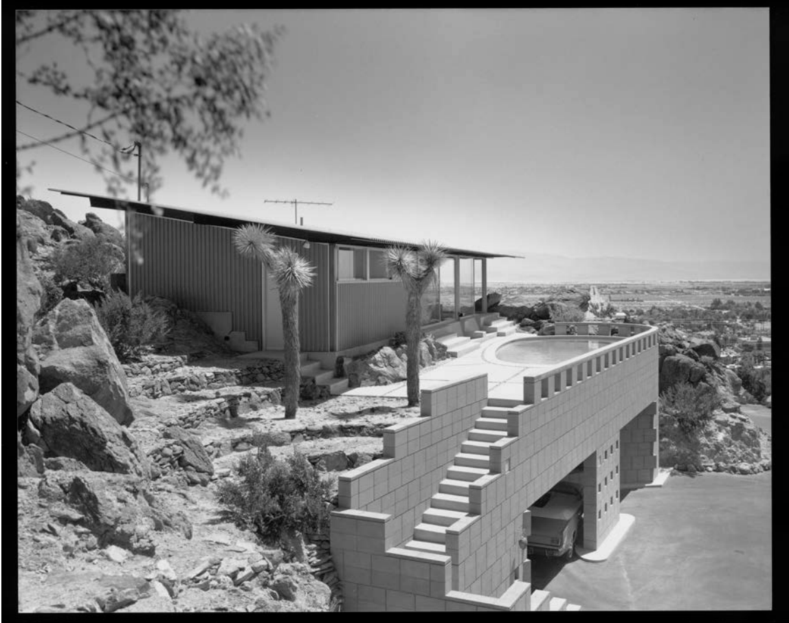
Figure 2. West and south elevations, looking northeast, 1965.
