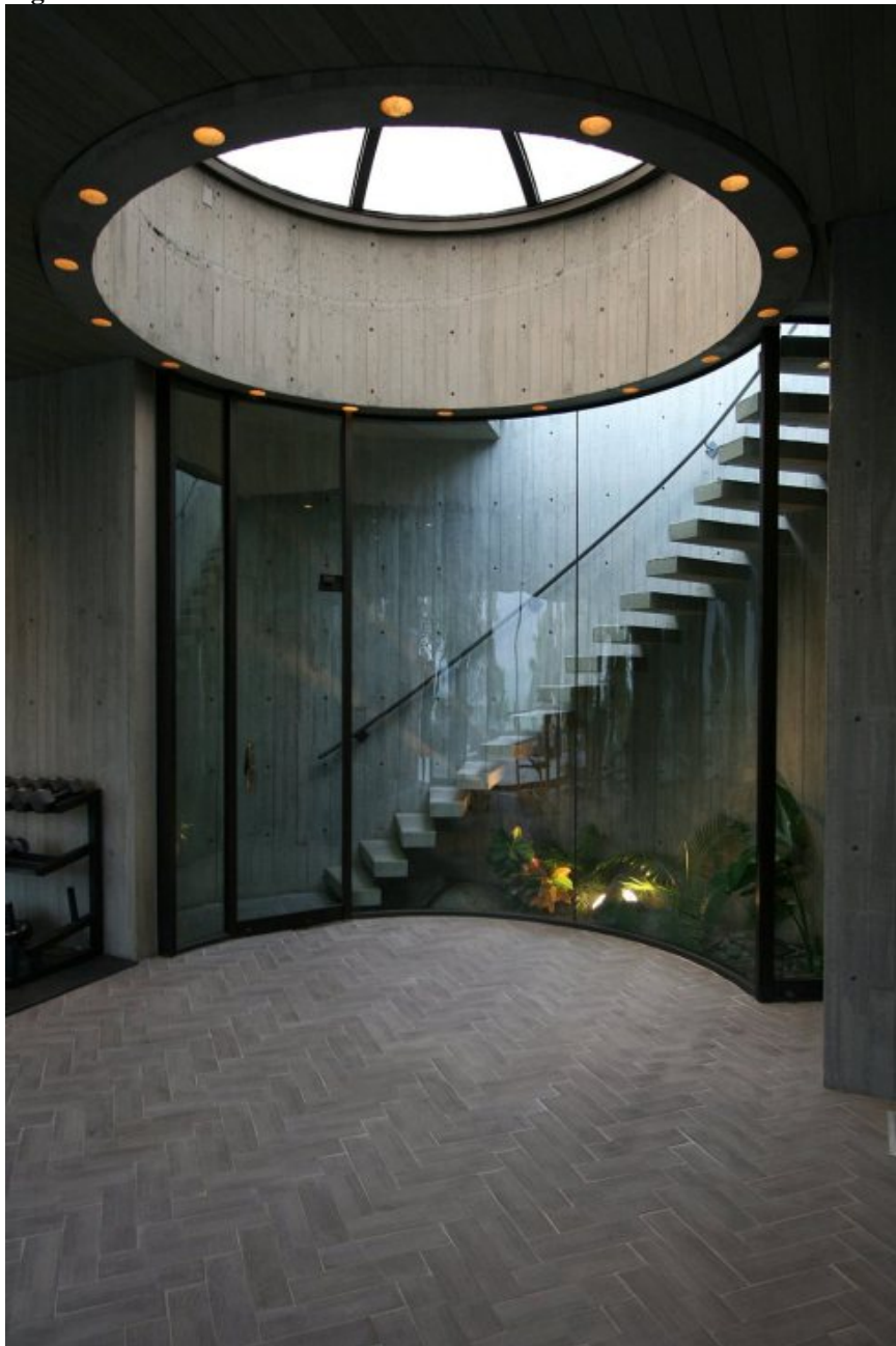
Interior detail of window system and stair well (Photo credit: Coronare Modestus Faust, photographed in 2011)
