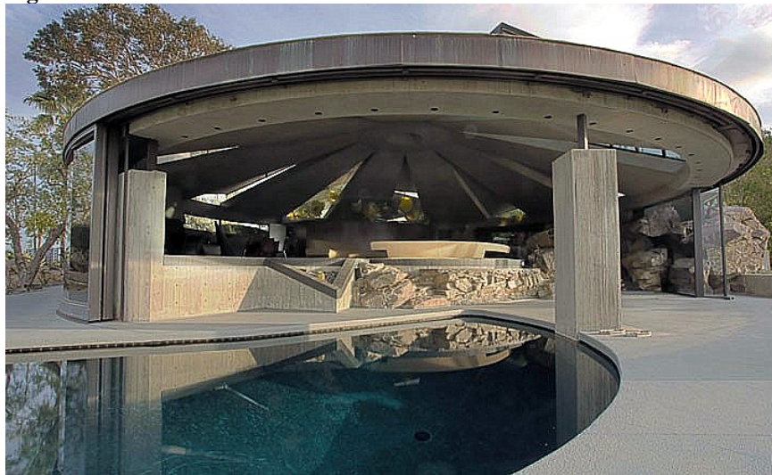
Detail of roof structure, facing south (Photo credit: Coronare Modestus Faust, photographed in 2011)
