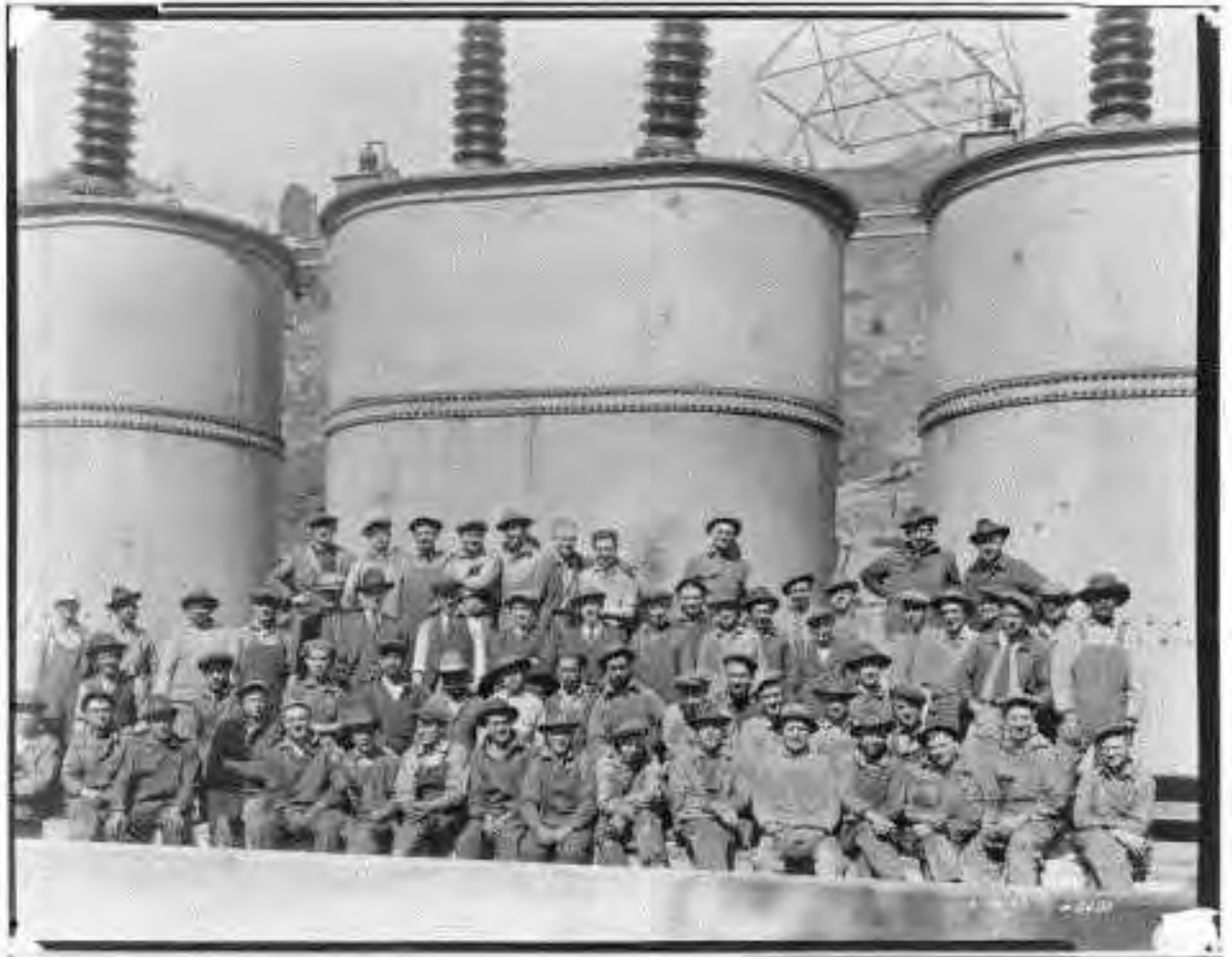
Figure 97: Eagle Rock Construction Gang, 1923. Image No. SCE-02-08480, Huntington Digital Library.
