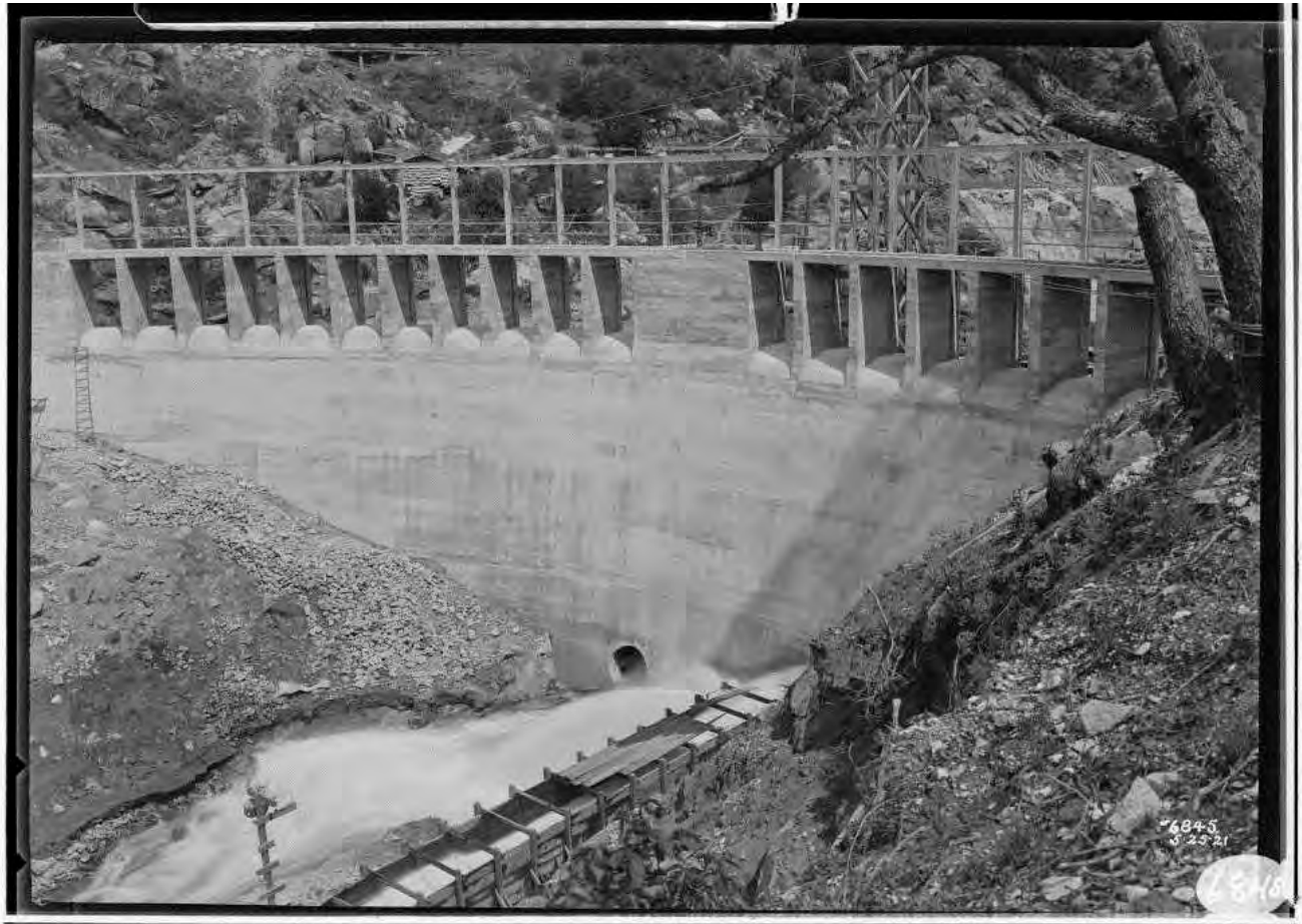
Figure 35: Dam No. 5 near completion, 1920. Image No. SCE-02-06845, Huntington Digital Library.
