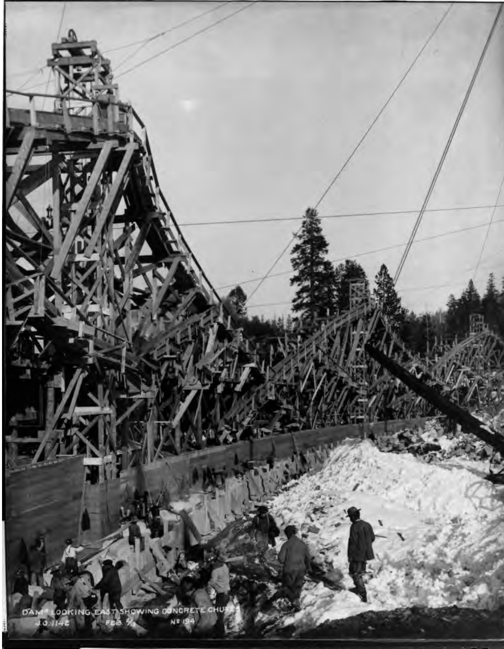
Figure 1: Huntington Lake Dam No. 1, circa February 1913.
