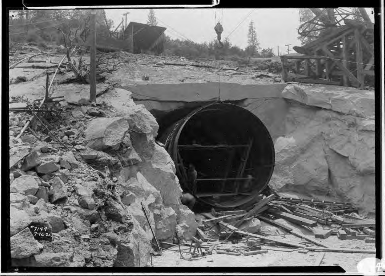
Figure 32: Tunnel No. 8 Outlet, to be connected to surge chamber, 1921. Image No. SCE-02-07144, Huntington Digital Library.
