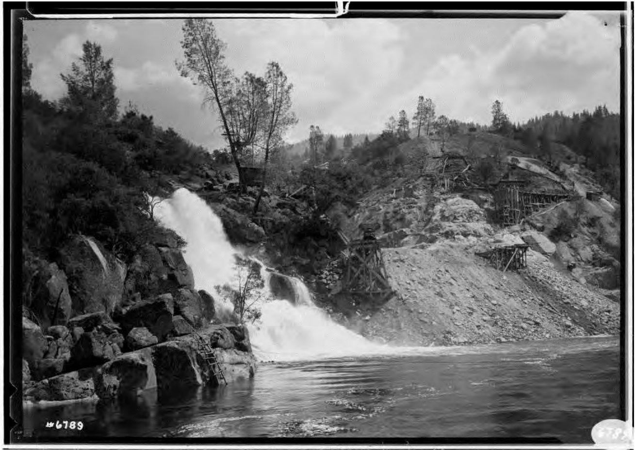
Figure 37: Excavation Site for Powerhouse No. 8, 1921. Image No. SCE-02-06789, Huntington Digital Library.
