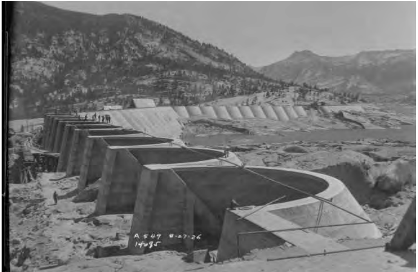
Figure 65: Florence Lake Dam construction, 1926. Image No. SCE-02-14085, Huntington Digital Library.
