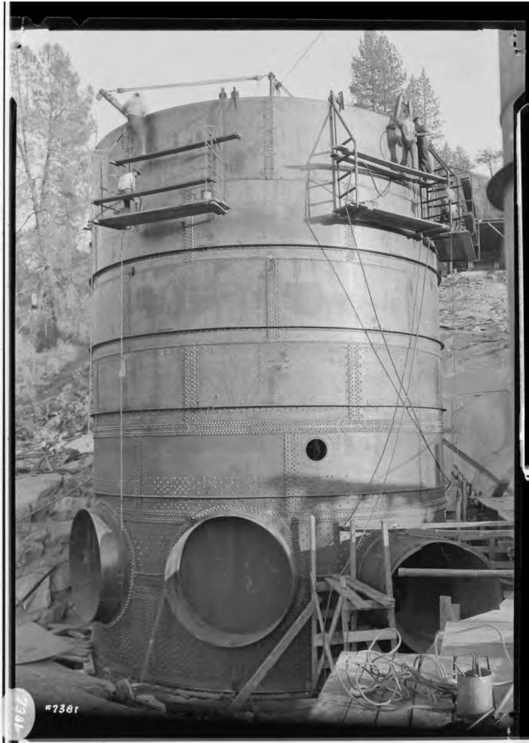
Figure 33: Powerhouse No. 8 Surge Tank, 1921. Image No. SCE-02-07381, Huntington Digital Library.
