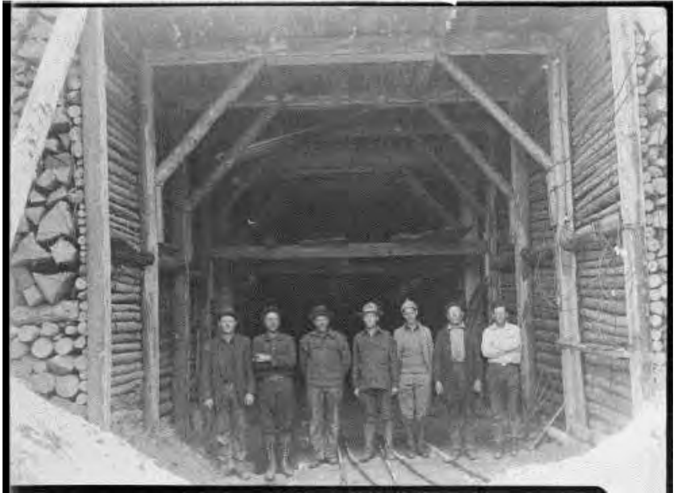
Figure 56: Portal of Florence/Ward Tunnel Adit 61, circa 1921. Image No. SCE-02-06807, Huntington Digital Library.
