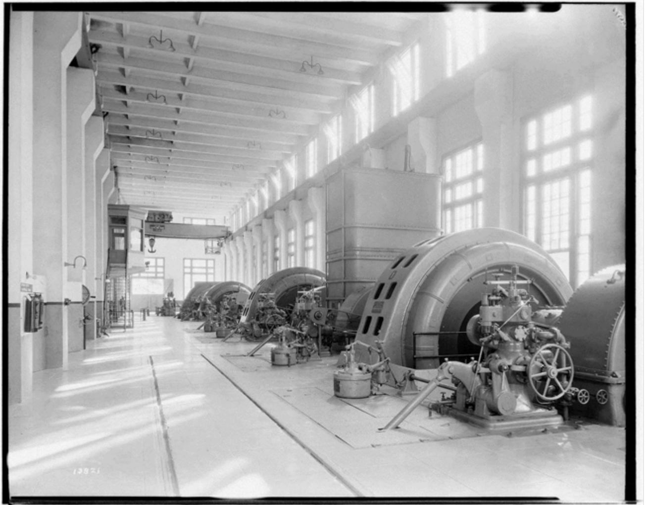
Figure 14: Interior of Powerhouse No.1 generator floor with 4 units installed, 1926. Image No. SCE-02-13821, Huntington Digital Library.
