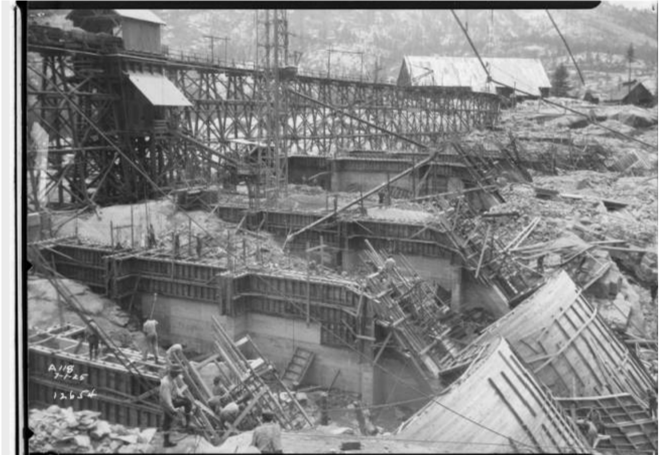
Figure 64: Florence Lake Dam construction, 1925. Image No. SCE-02-12654, Huntington Digital Library.
