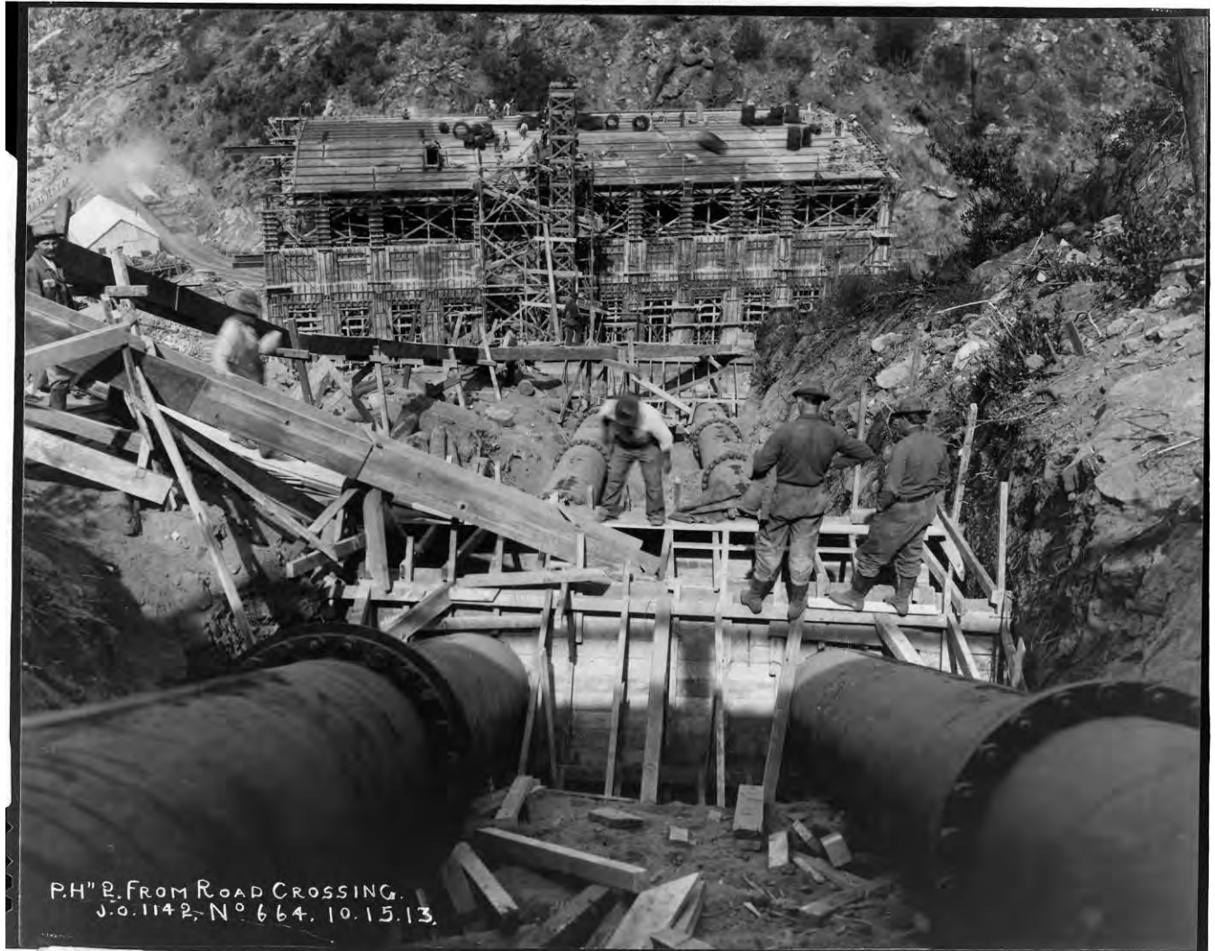
Figure 23: Penstocks for Powerhouse No. 2 looking toward the still-incomplete powerhouse, 1913. Image No. SCE-12-00044, Huntington Digital Library.
