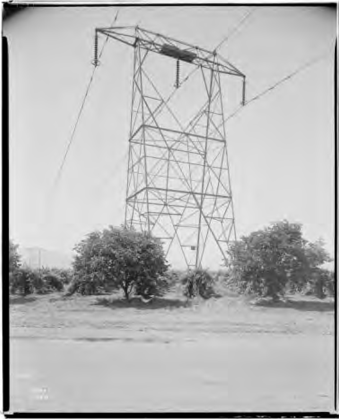
Figure 94: Vincent Transmission Line Tower, 1937. Image No. SCE-02-19979, Huntington Digital Library.
