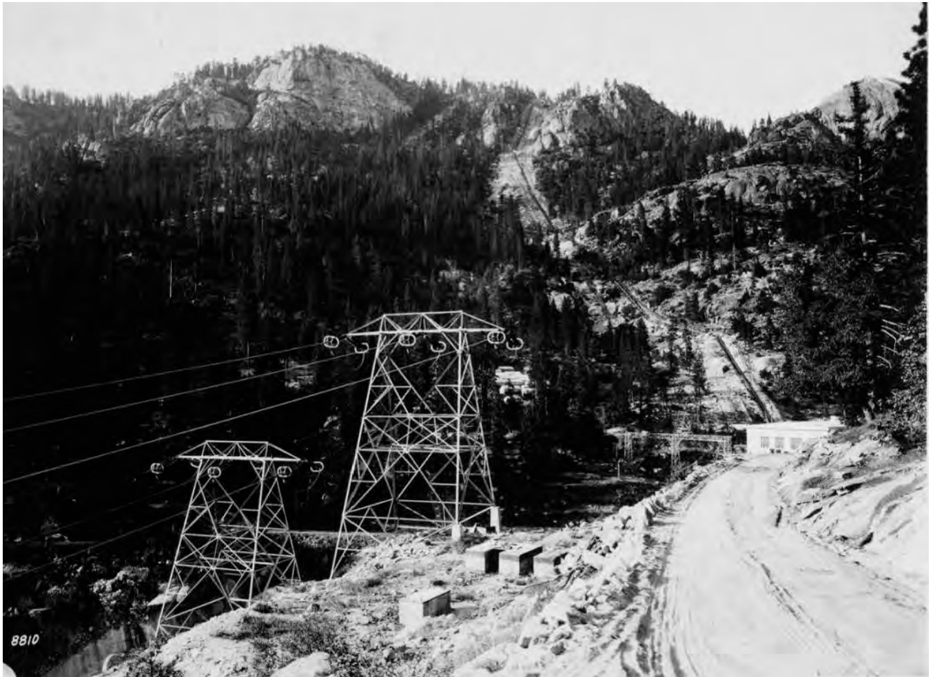
Figure 89: Big Creek East and West Transmission Lines, 1923. Image No. SCE-02-08810, Huntington Digital Library.
