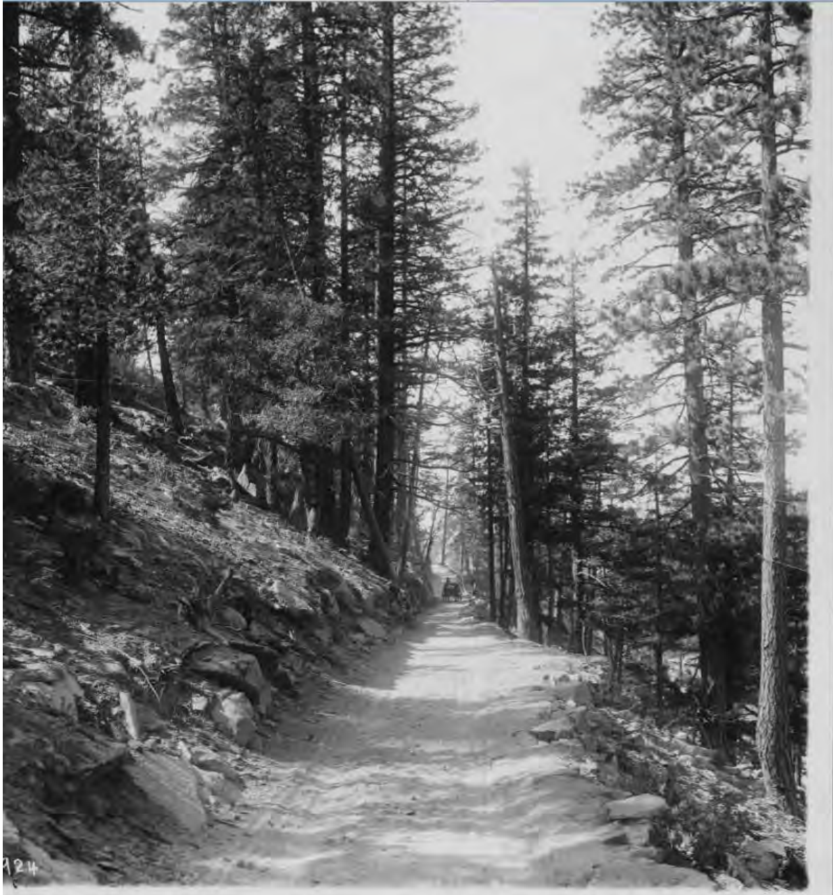
Figure 108: SJ&E grade under construction, 1912. Pacific Light and Power Corporation, 13-Vol. 018, Huntington Digital Library.
