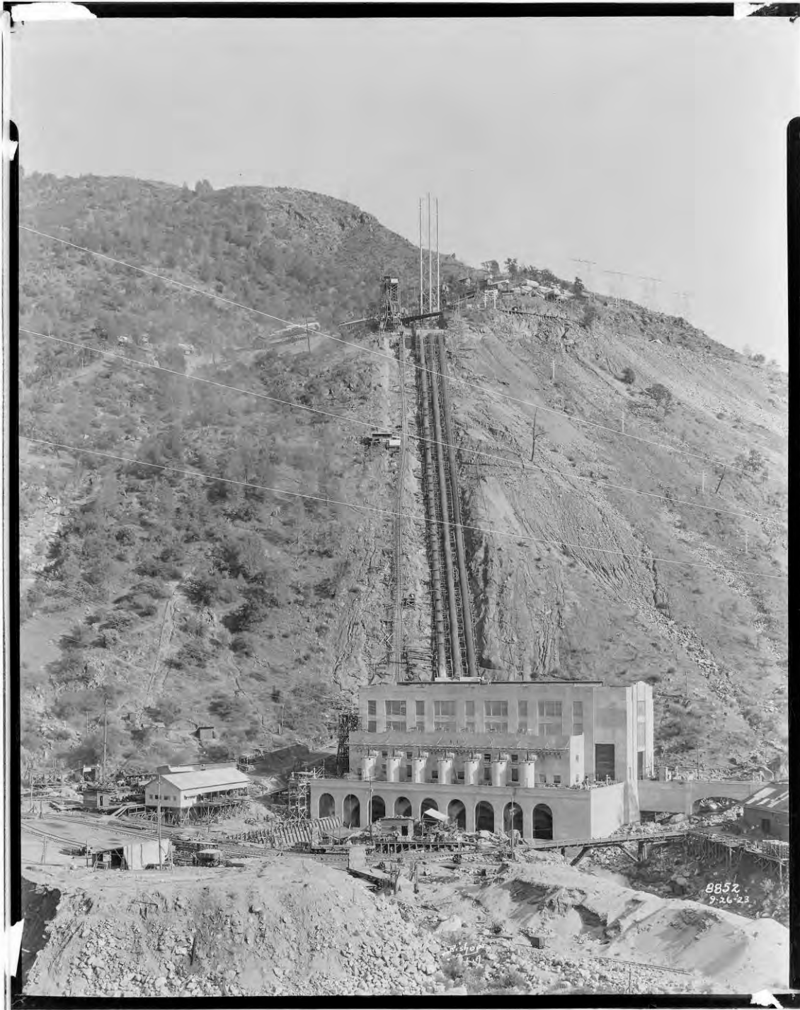
Figure 51: Powerhouse No. 3 and Penstocks, 1923. Image No. SCE-02-08852, Huntington Digital Library.
