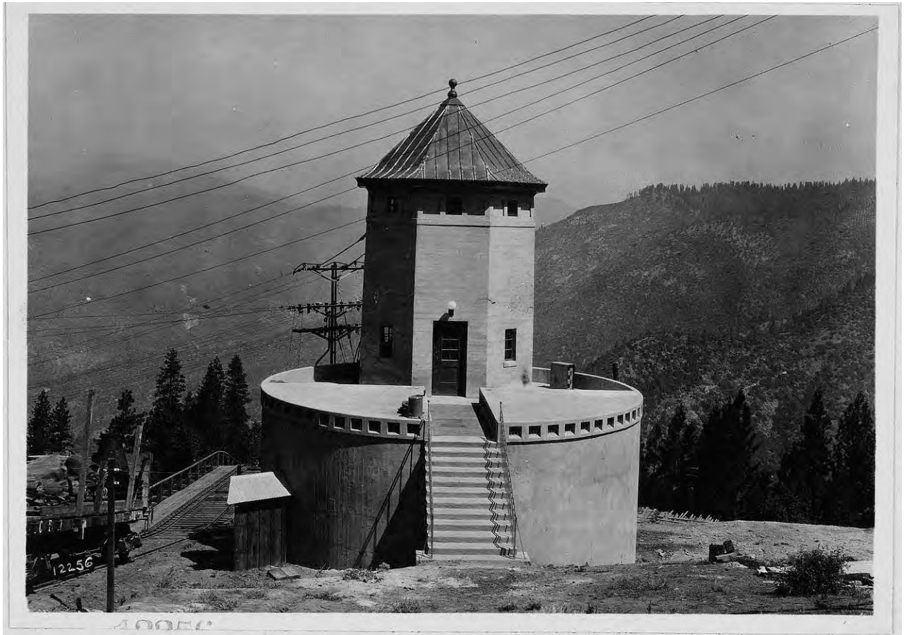
Figure 20: Tunnel No.2 Flowline Gate House (surge chamber) located at West Portal (termination of Tunnel No. 2), 1924.
