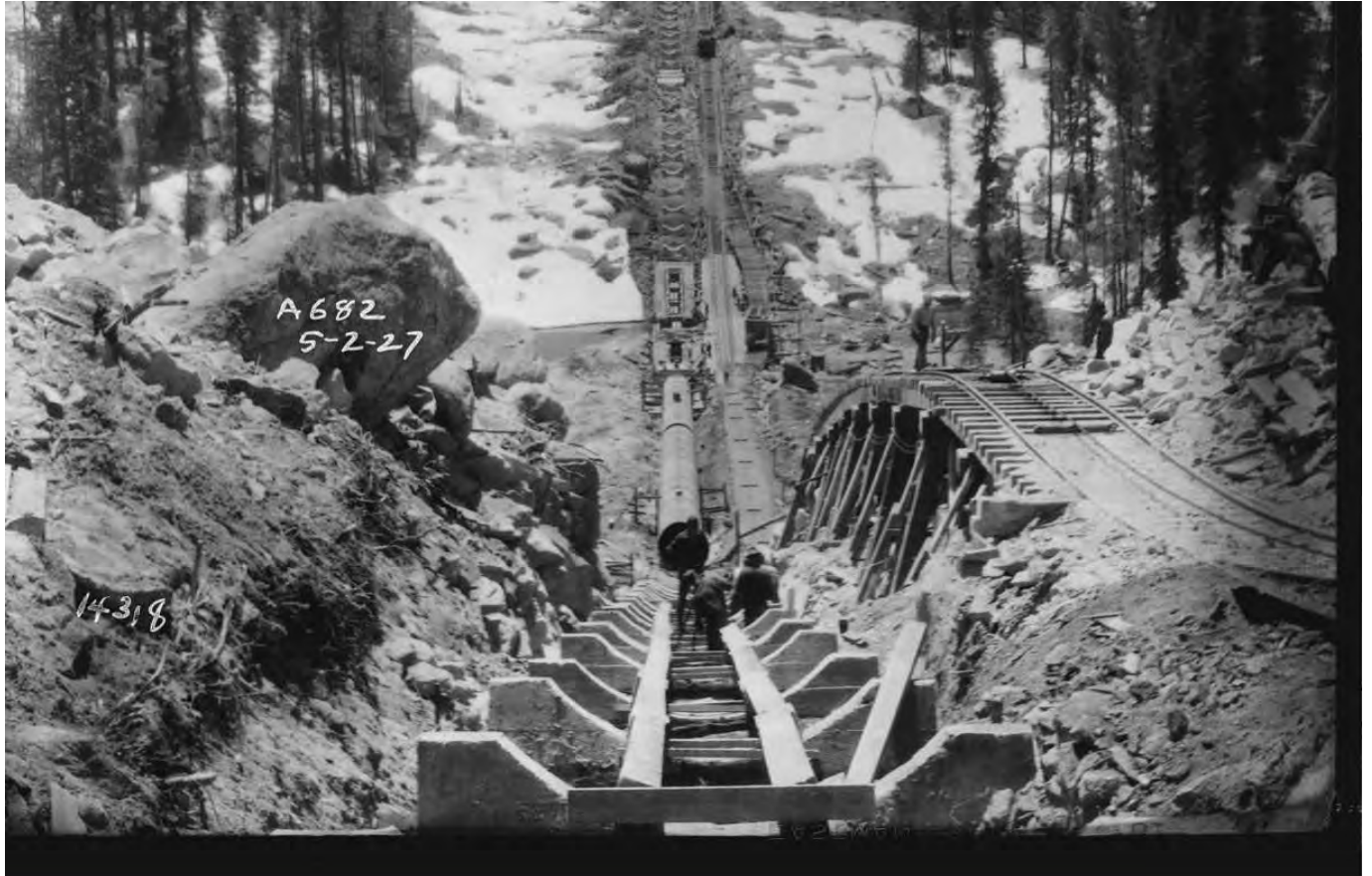
Figure 83: Tunnel No. 7 Flowline construction, 1927. Image No. SCE-02-14318, Huntington Digital Library.
