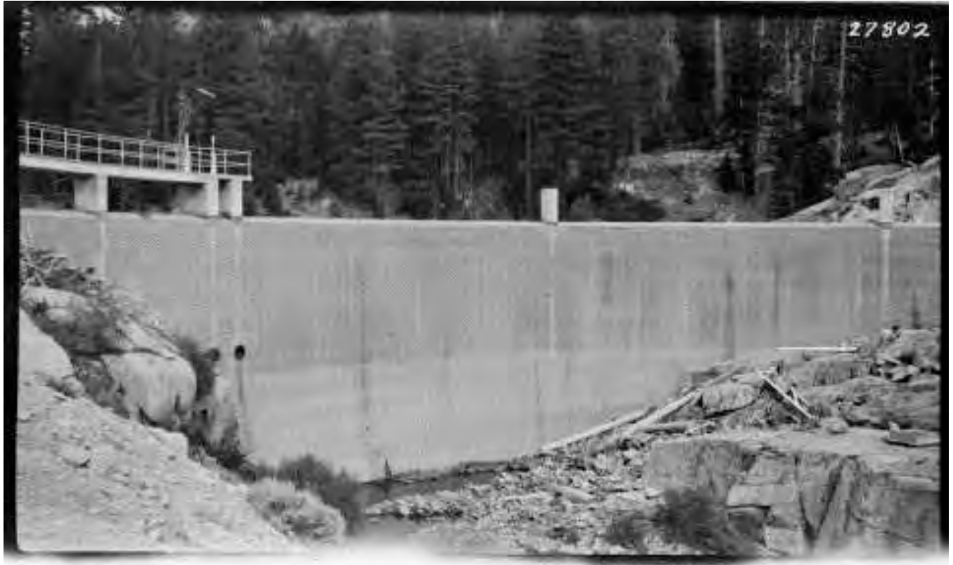
Figure 71: Bear Creek Diversion Dam, 1947. Image No. SCE-02-27802, Huntington Digital Library.
