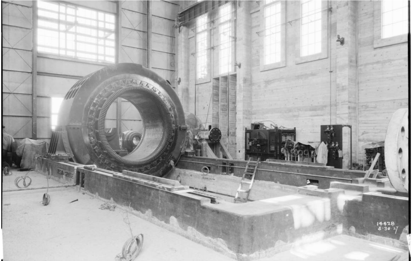
Figure 105: Rector Substation Interior, Frequency Changer being placed, 1927. Image No. SCE-02-14428, Huntington Digital Library.
