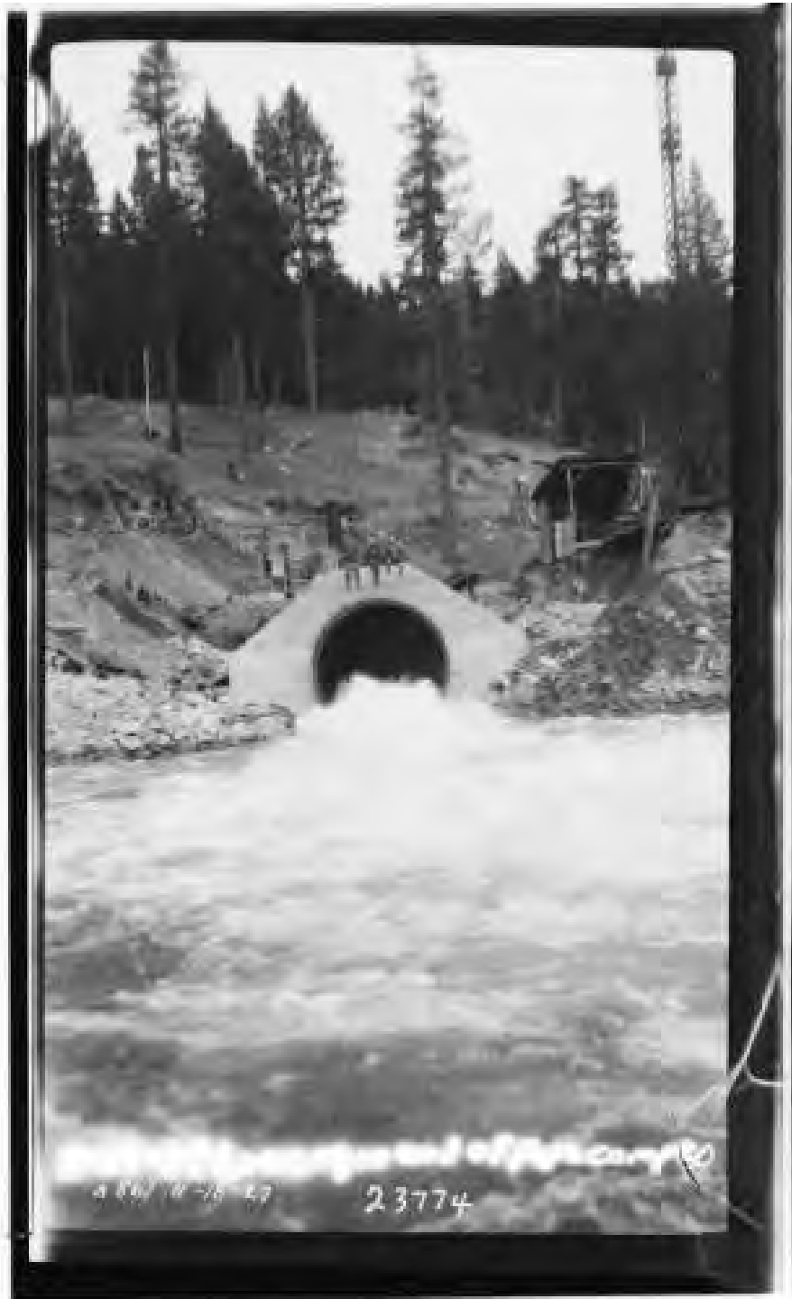
Figure 59: Outlet of Florence/Ward Tunnel, 1927. Image No. SCE-02-23774, Huntington Digital Library.
