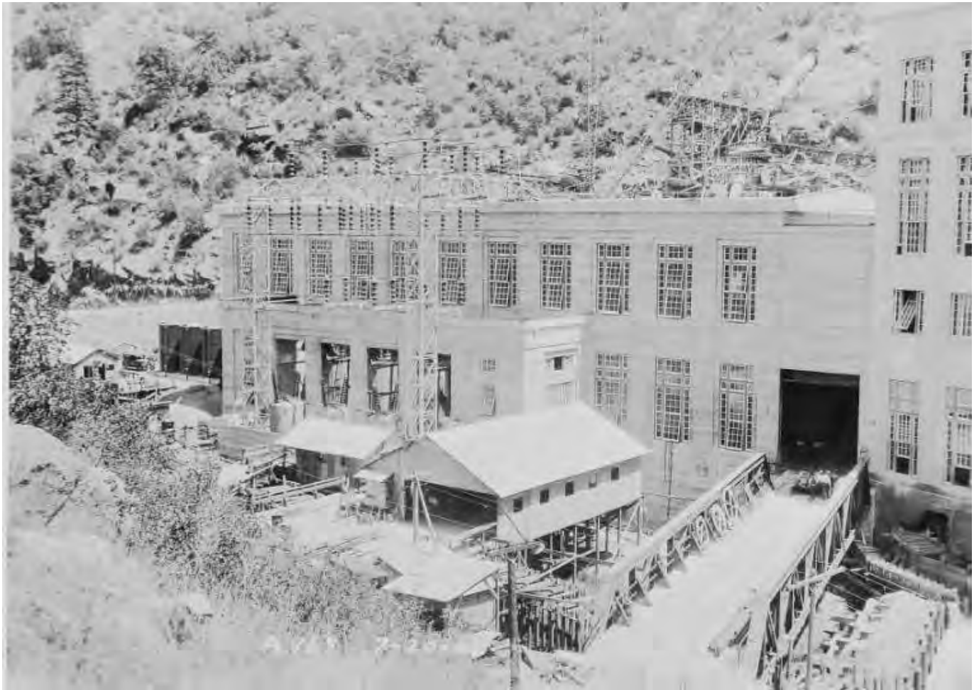
Figure 85: Powerhouse No. 2A under construction, 1928. Image No. SCE-02-15904, Huntington Digital Library.
