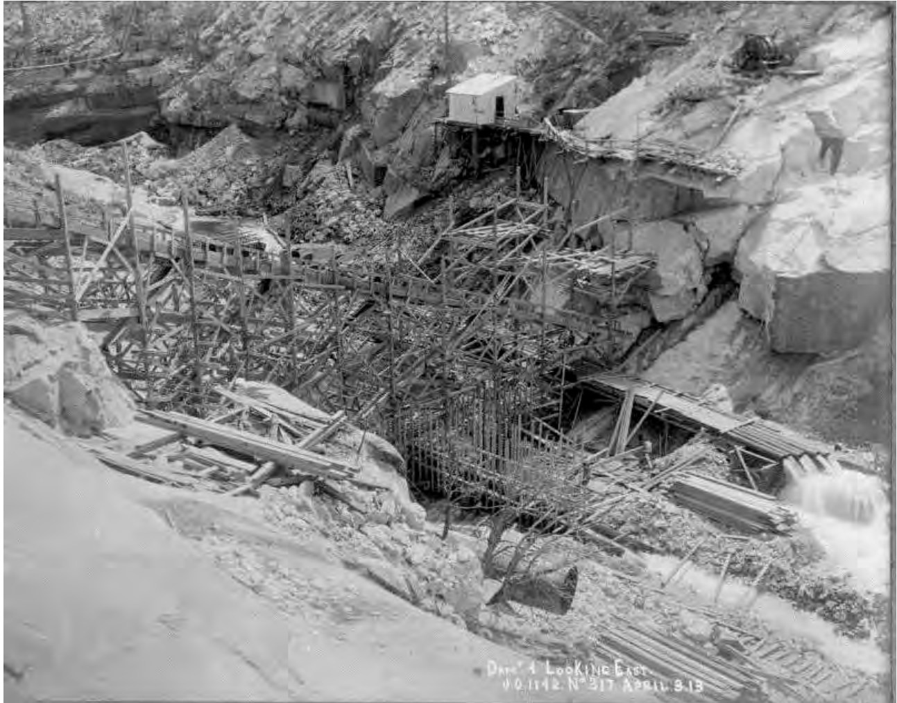
Figure 17: Construction of Dam No. 4, 1913. Image No. SCE-10-00008, Huntington Digital Library.
