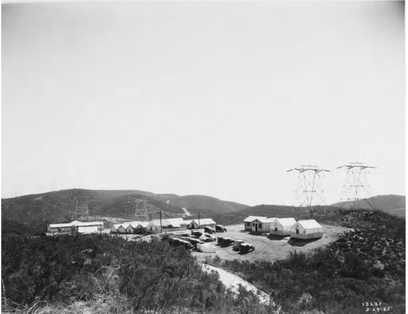
Figure 92: Vincent Transmission Line at site of Gould Substation, 1925. Image No. SCE-02-13221, Huntington Digital Library.
