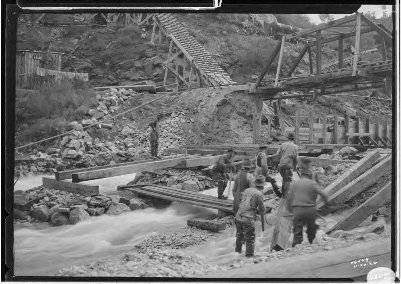
Figure 34: Construction on Dam No. 5, 1920. Image No. SCE-02-06509, Huntington Digital Library.
