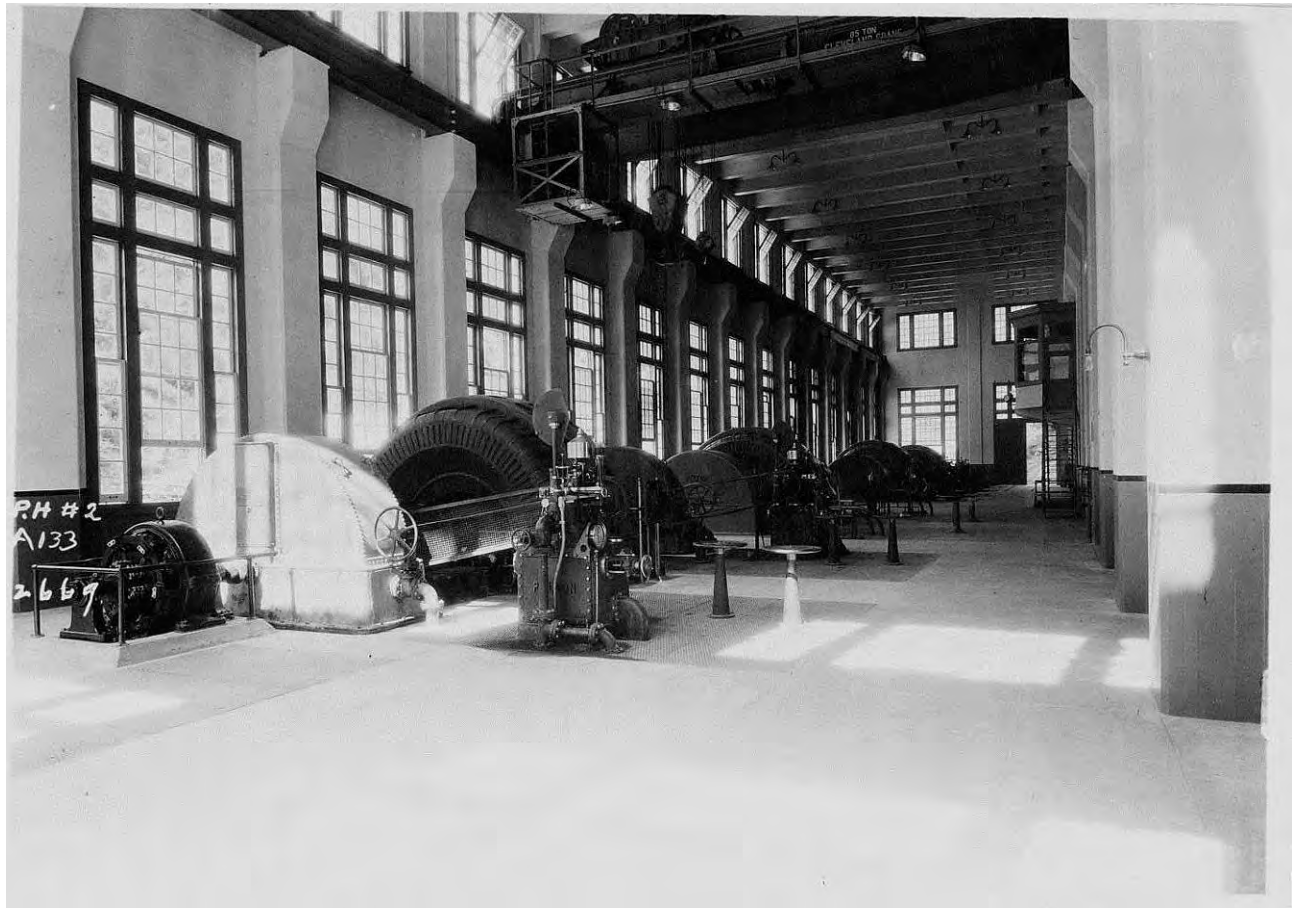
Figure 25: Interior of generator floor for Powerhouse No. 2, 1925. Image No. SCE-02-12669, Huntington Digital Library.
