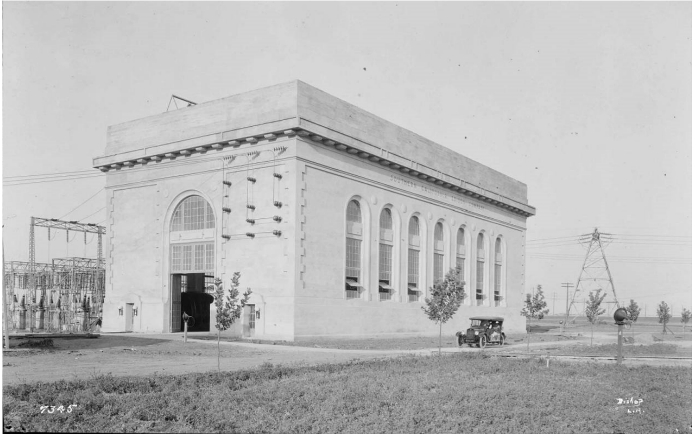
Figure 101: Vestal Substation, with Big Creek East and West Transmission Lines, 1921. Image No. SCE-02-07345, Huntington Digital Library.
