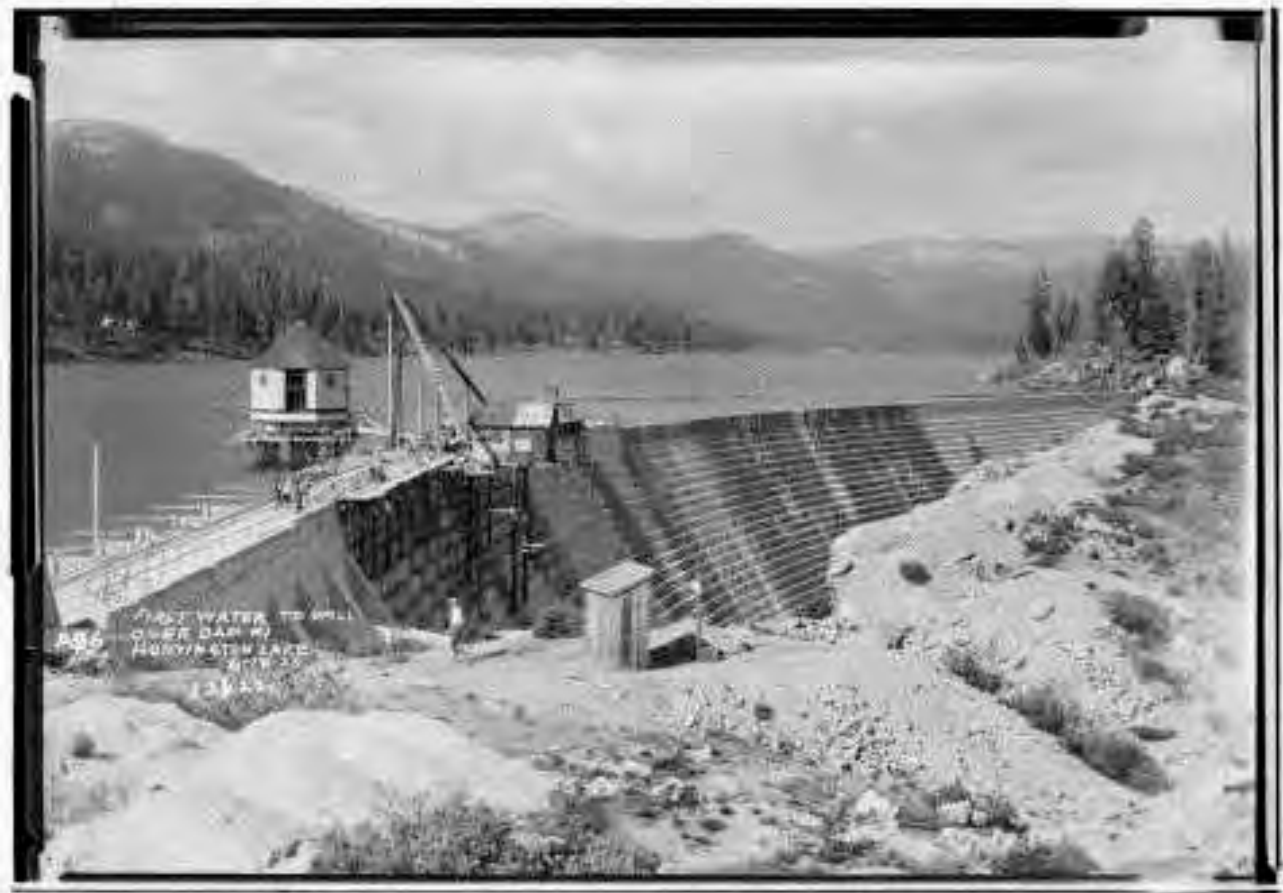
Figure 2: Huntington Lake Dam No. 1, 1925. First water to spill over dam from water conveyed by Florence (Ward) Tunnel. Image No. SCE-02-12622, Huntington Digital Library.
