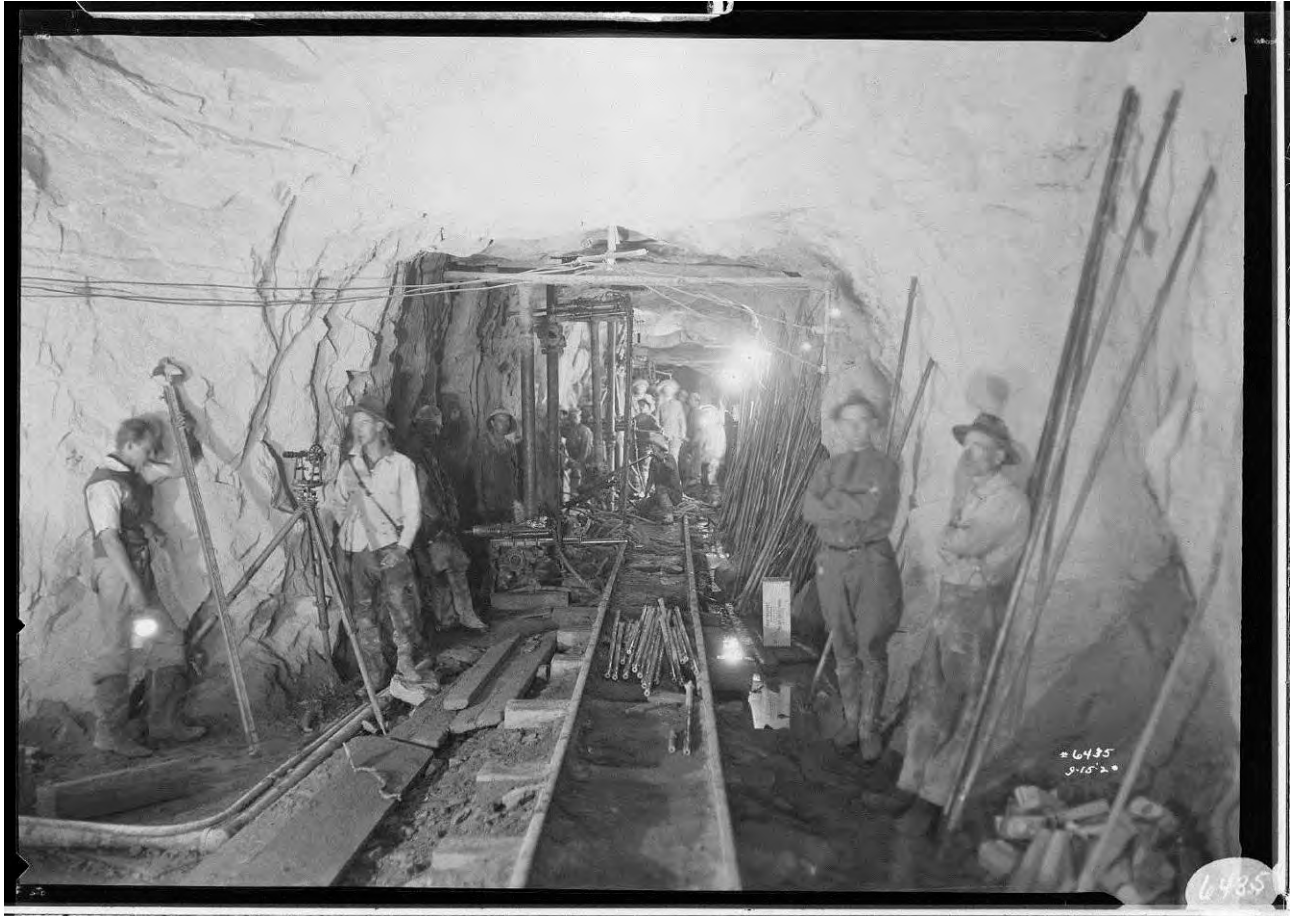
Figure 31: Tunnel No. 8 near Camp 31, depicting crew expanding pioneer bore to full tunnel width, 1920. Image No. SCE-02-06435, Huntington Digital Library.
