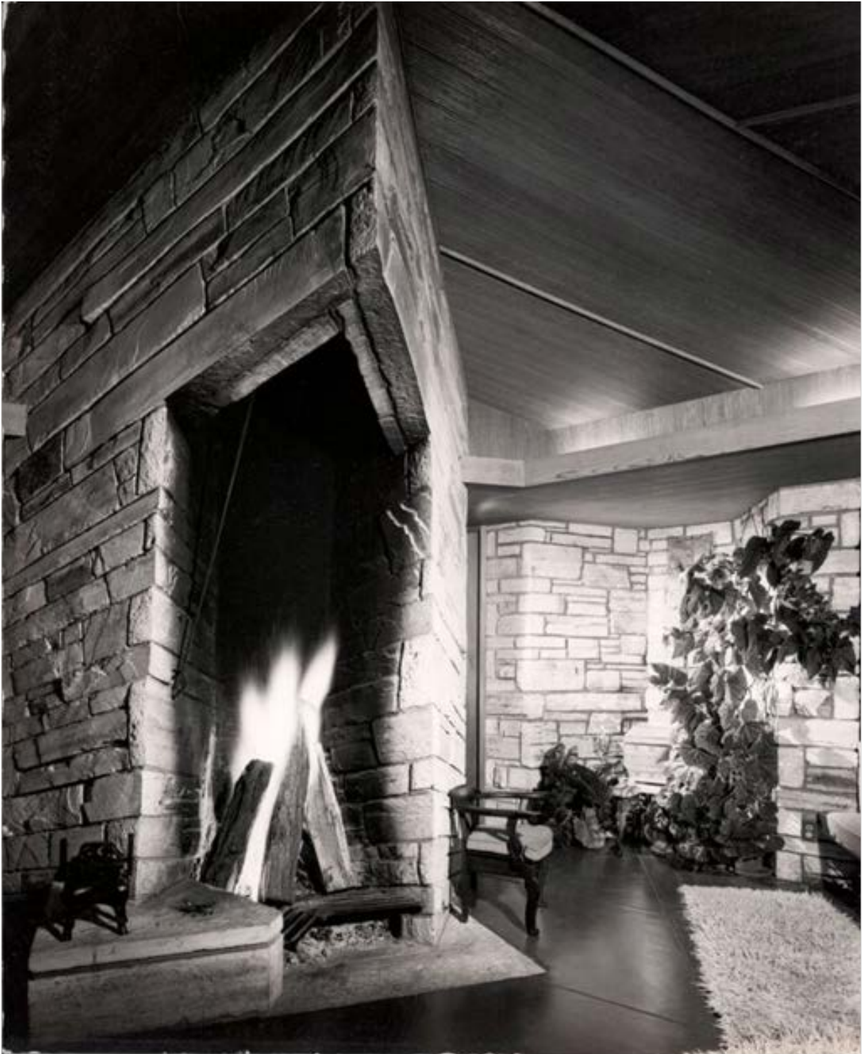
Figure 10 Circa 1954 photograph of Walker House fireplace
