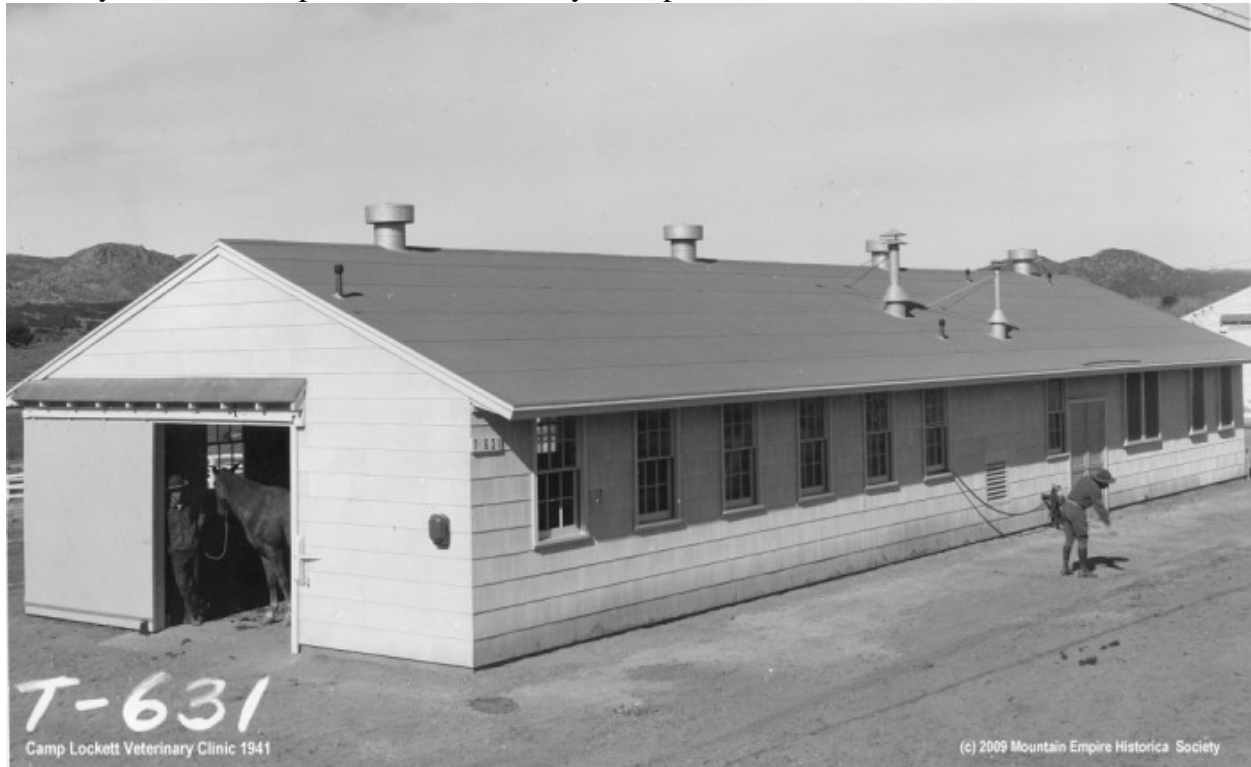
Figure 20. Type C-6 veterinary clinic, surgical, Series 700-272 drawing, Building T-631, Camp Lockett, San Diego County, California, 1941. This is the only other example of a Type C-6 building that Fort Ord SVH researcher Krenzelok was able to locate in the United States. Photo courtesy Mountain Empire Historical Society, Campo, California. From Krenzelok.
