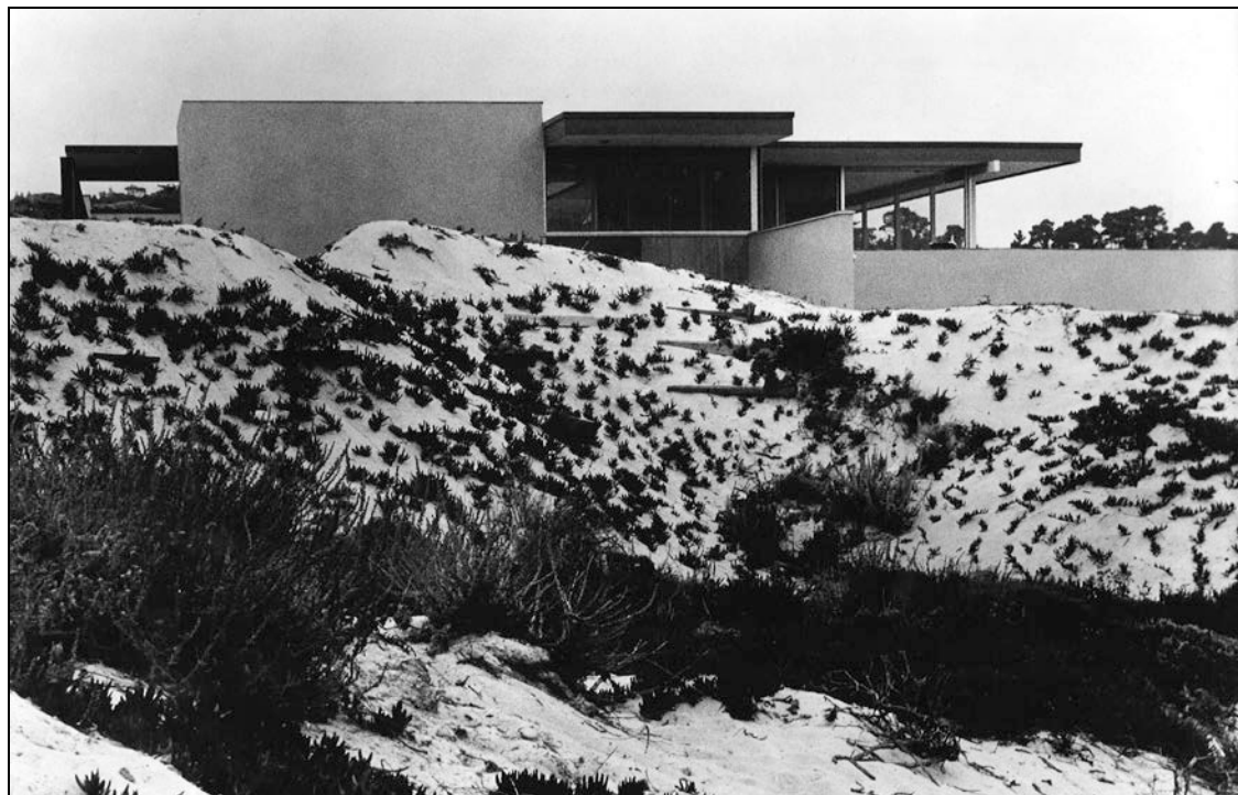
Figure A. Looking south at north elevation.
