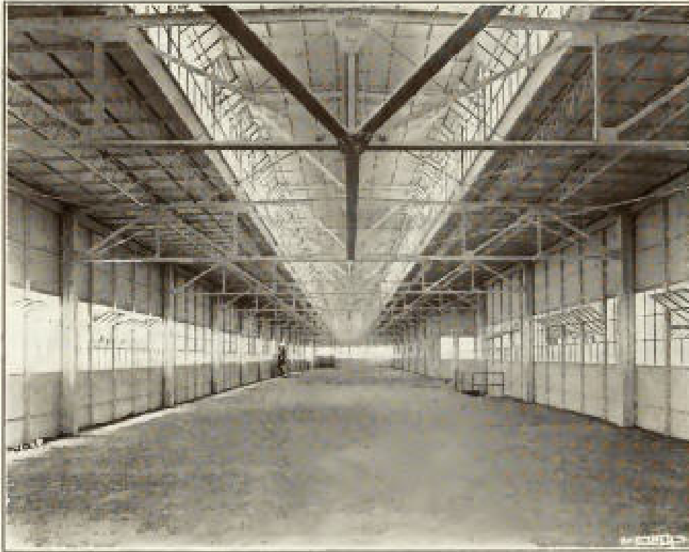
Showing Wood Block Floor, Second Floor of New Factory Building.
