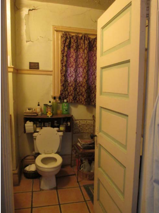
25 of 30. Interior: Hollywood School for Girls second floor bathroom, view north
