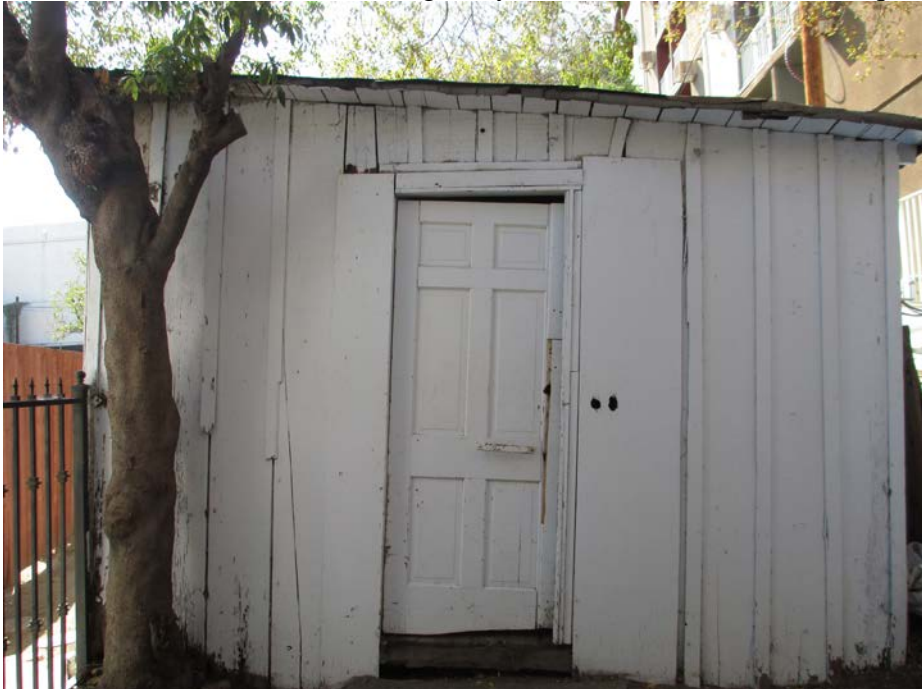
28 of 30. Exterior: Shed used originally as classroom and teachers' quarters, view west
