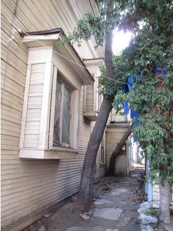
15 of 30. Exterior: North façade, Hollywood School for Girls, view west
