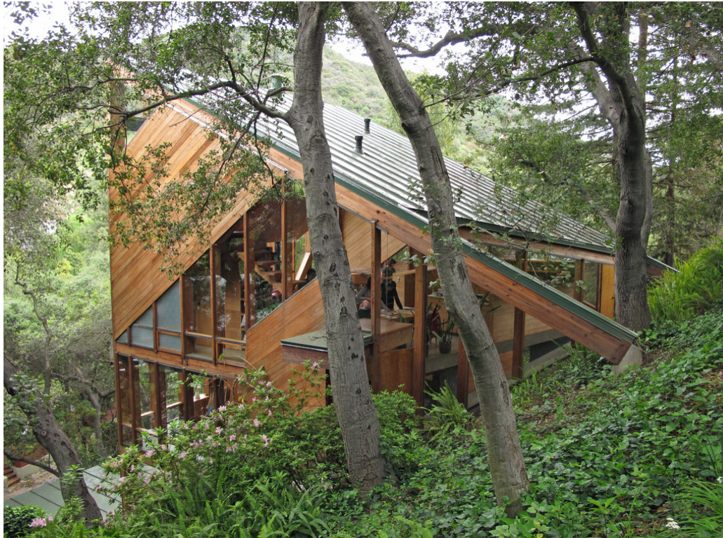
View of west and south façades. (Photo credit: Shelly White, date of photograph unknown)
