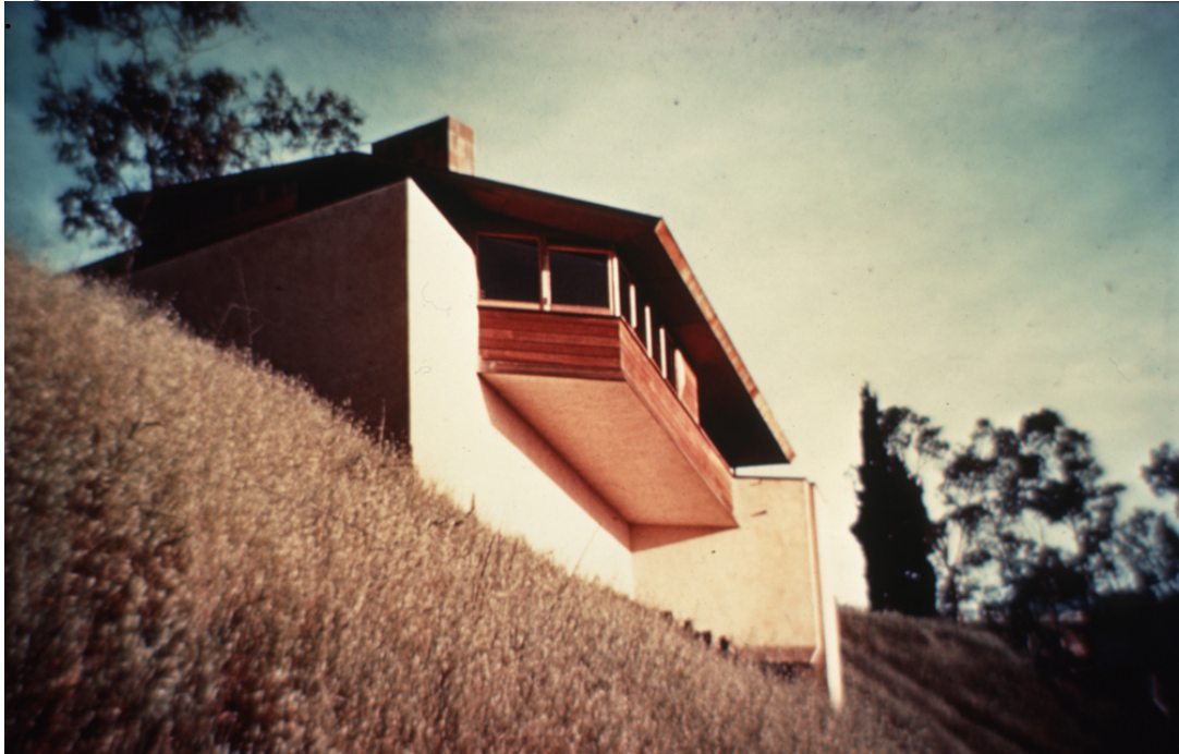
View of north and west façades, facing southeast (© The John Lautner Foundation, courtesy of Frank Escher, date of photograph unknown)
