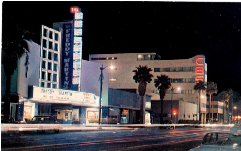
Figure 15. Context view along Sunset Boulevard, view facing northeast, c. 1950. Source: Hollywood Heritage
