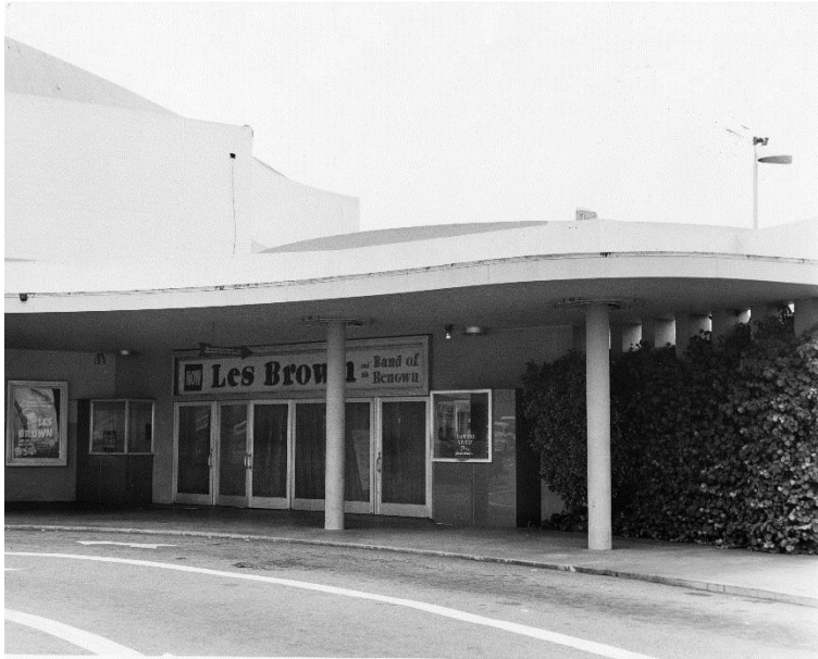
Figure 14. Detail view of west façade entrance, view facing east, 1950. Source: Bison Archives (Marc Wanamaker)
