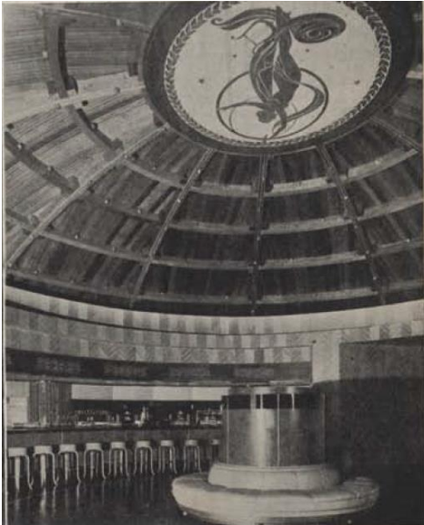
Figure 8. Detail of dancehall ceiling and ceiling medallion, 1940. Source: Southwest Builder and Contractor , December 20, 1940
