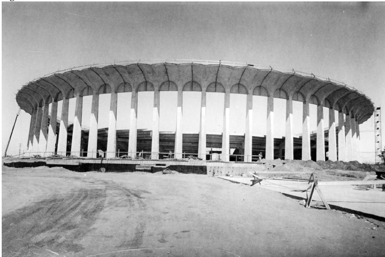
Forum under construction, 1967. Source: Forum archive.
