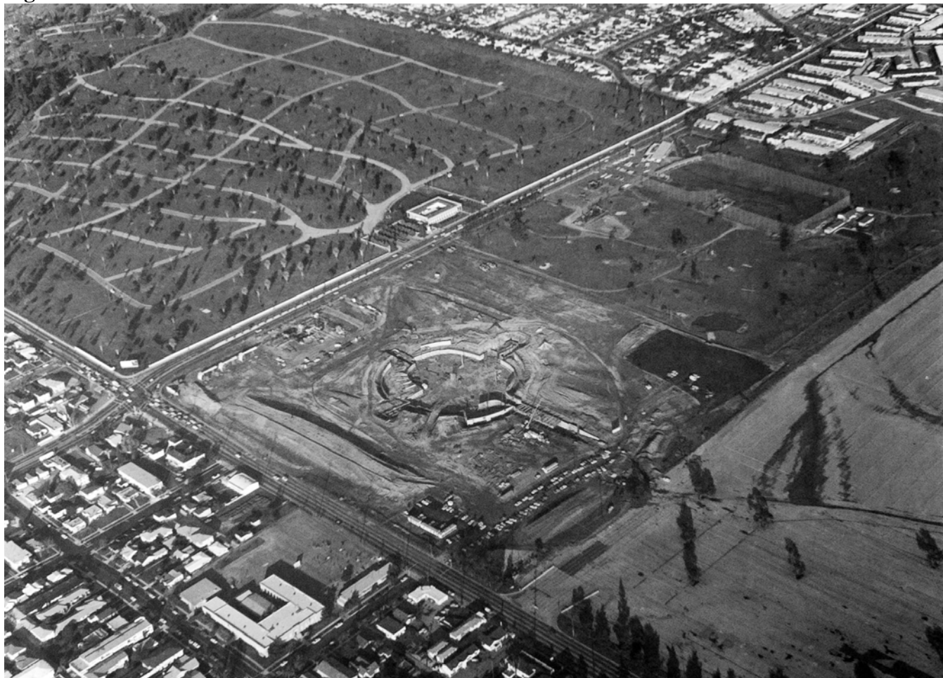
Aerial view of construction site, 1967. Source: Forum archive.
