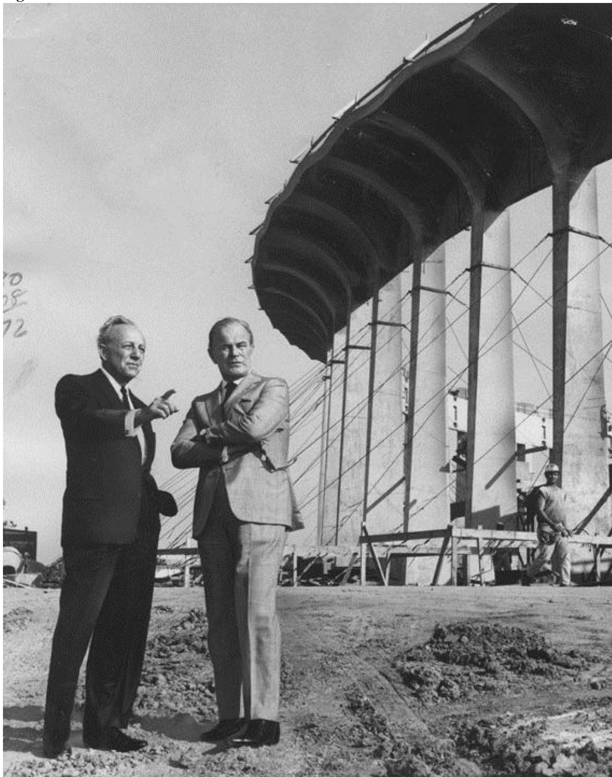
Jack Kent Cooke and Charles Luckman during construction of the Forum, 1967. Source: Los Angeles Public Library.
