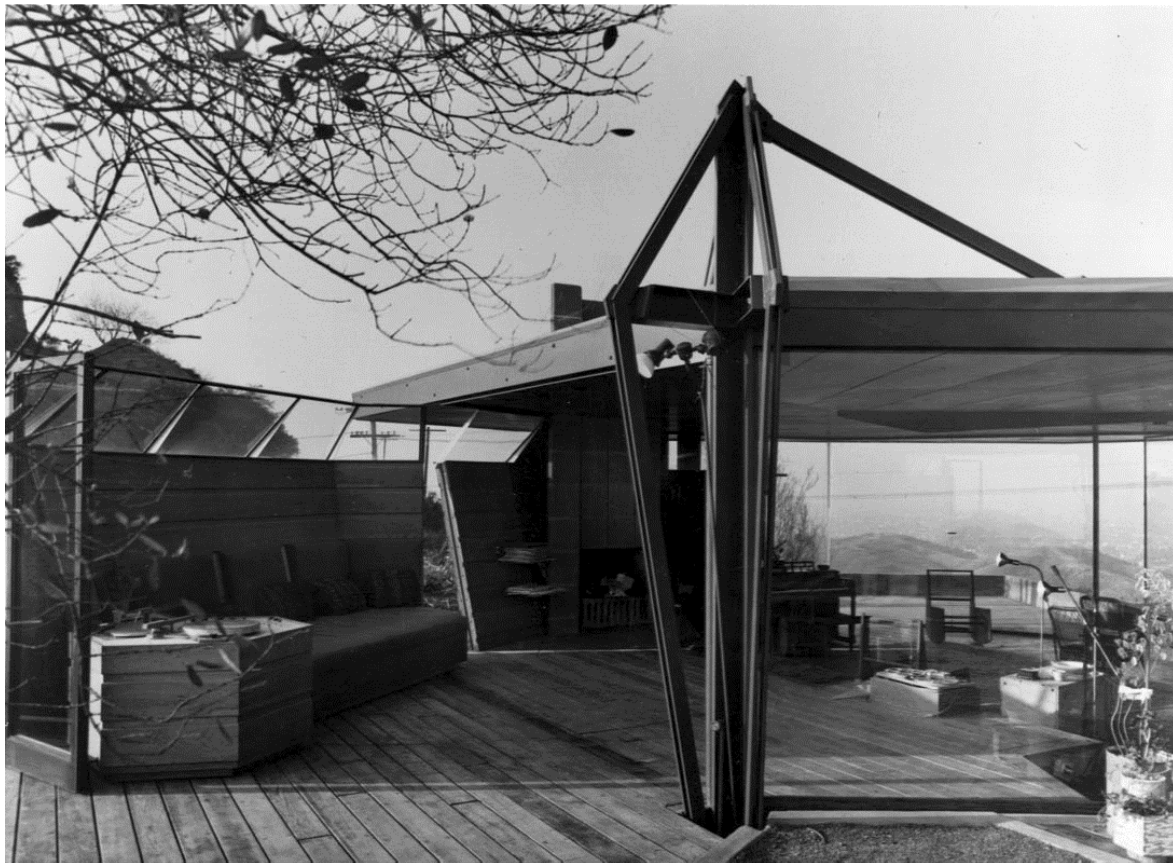
View of pivoting wall and roof support on south façade, facing northwest (© The John Lautner Foundation, courtesy of Frank Escher, date of photograph unknown)
