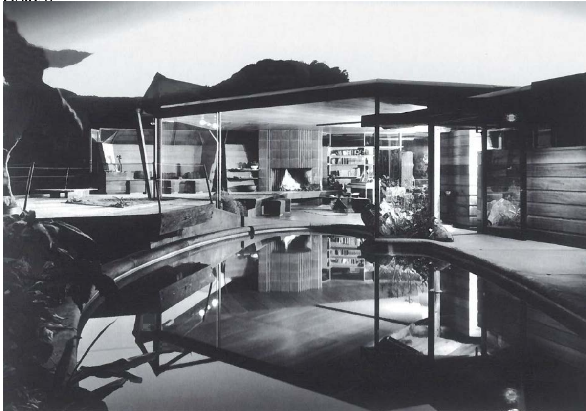
View of south façade, facing northwest (Photo credit: Don Higgins, Lautner by Barbara-Ann Campbell-Lange, date of photograph unknown)
