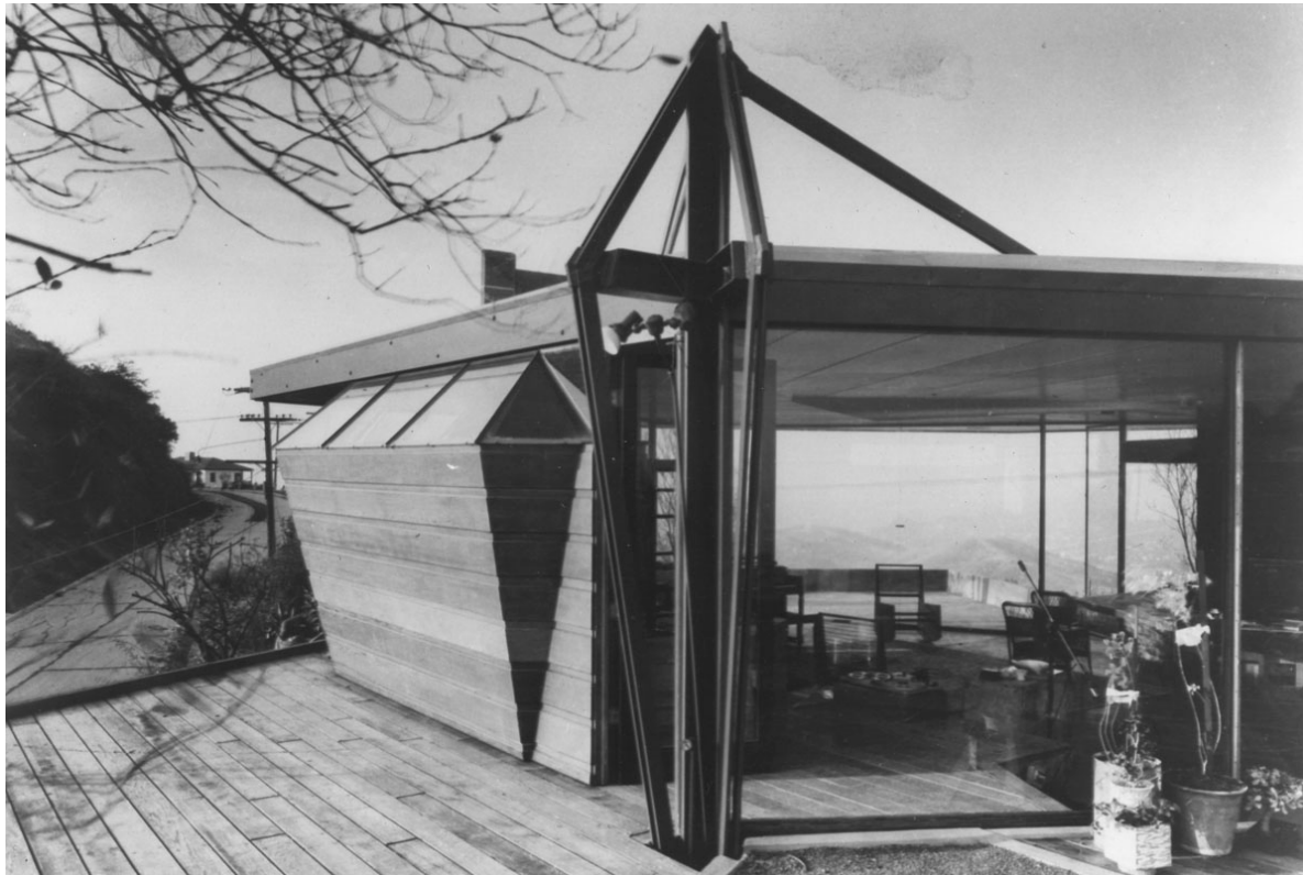
View of pivoting wall and roof support on south façade, facing northwest (© The John Lautner Foundation, courtesy of Frank Escher, date of photograph unknown)
