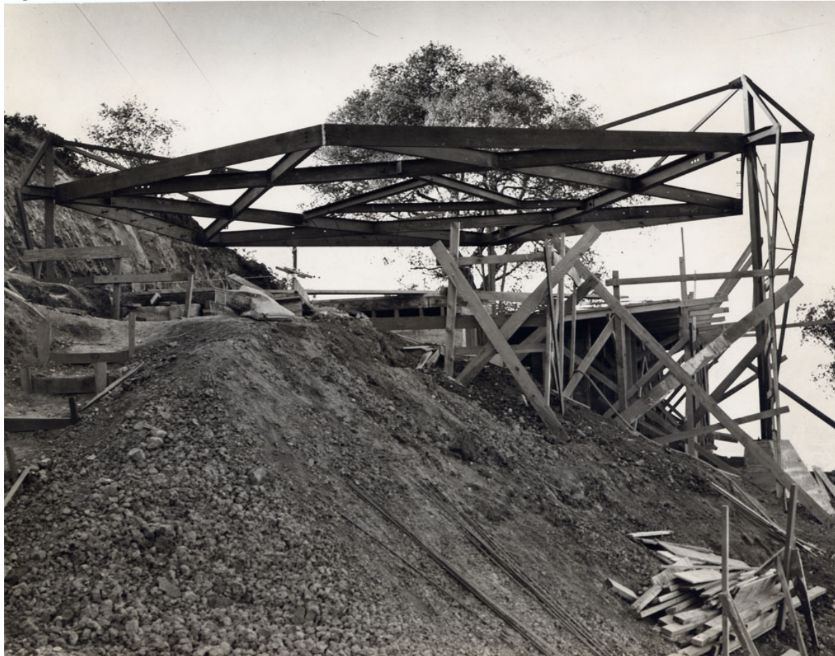
View of prefabricated roof structure, facing southeast (© The John Lautner Foundation, courtesy of Frank Escher, 1948)
