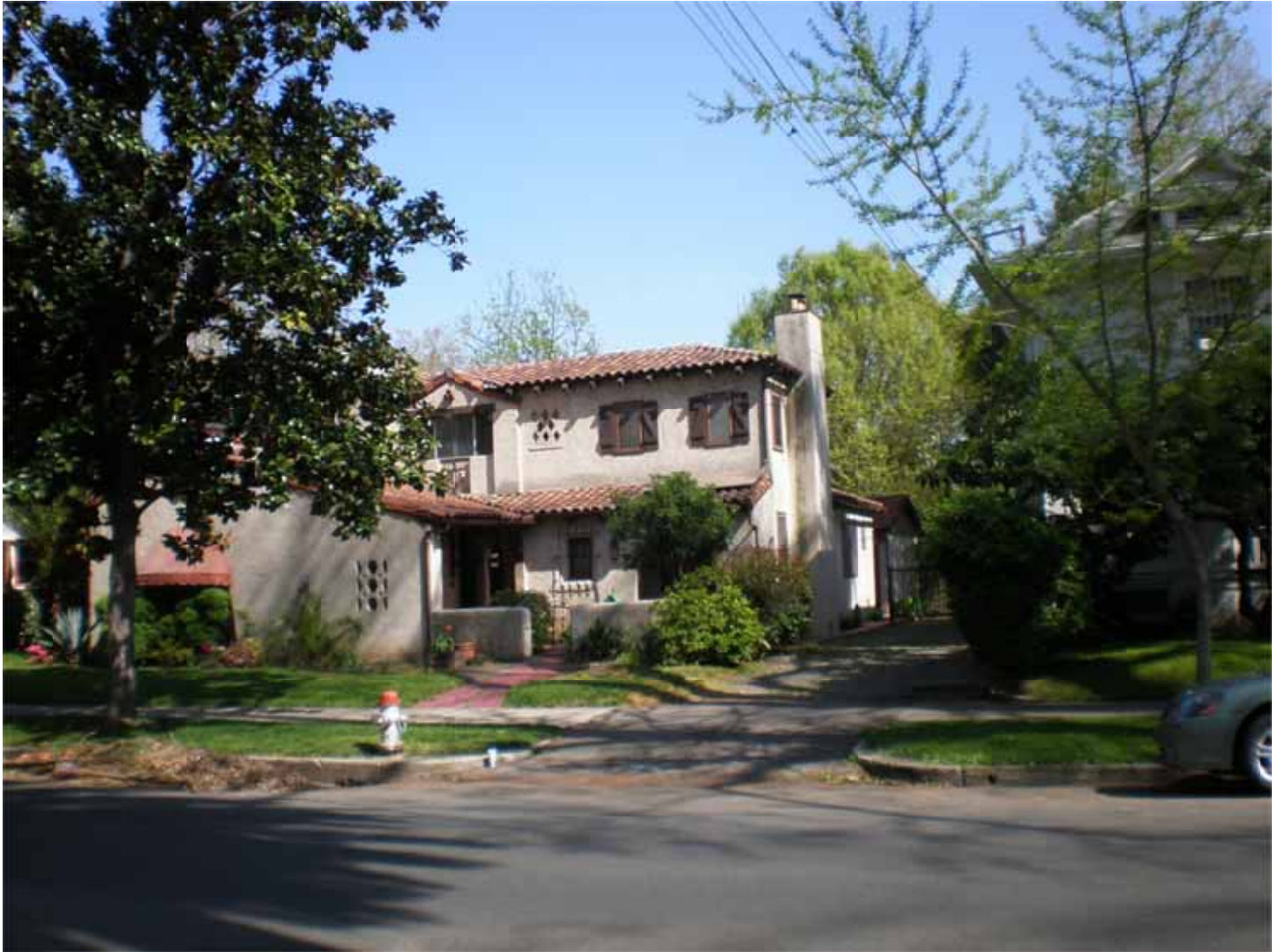
California_Sacramento_Boulevard Park_0018 Clarence H. Smith House, Spanish Colonial Revival residence, 615 21 st Street, facing east
