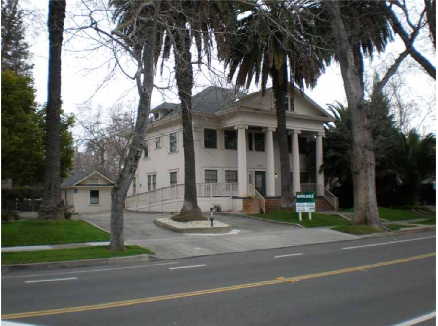
California_Sacramento_Boulevard Park_0023 George Smith House, Classical Revival residence and outbuilding, 2015-2013 H Street, facing northeast
