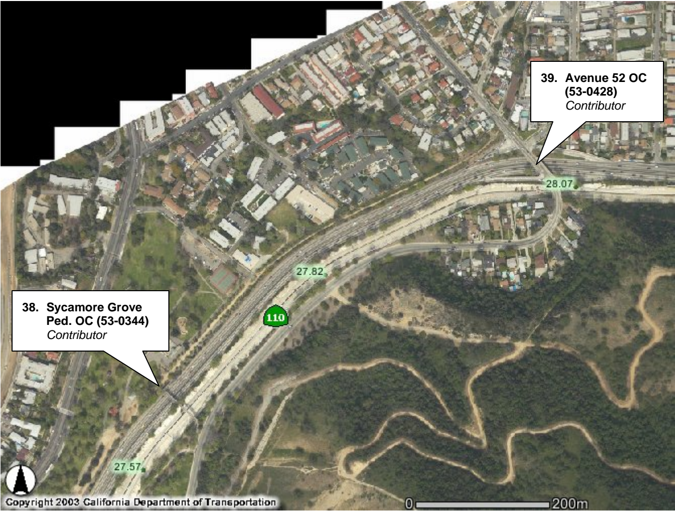
Arroyo Seco Parkway Historic District Segment H
