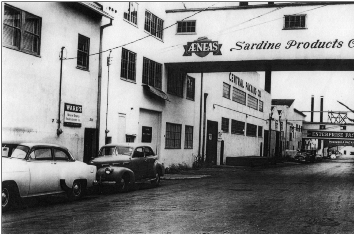
Figure 5. 1946 view of west façade of Aeneas Cannery building and crossover shortly after completion. Note that the name on the crossover reads, “Aeneas Sardine Products Company.” (Courtesy of the Pat Hathaway Collection of Historical Views)
