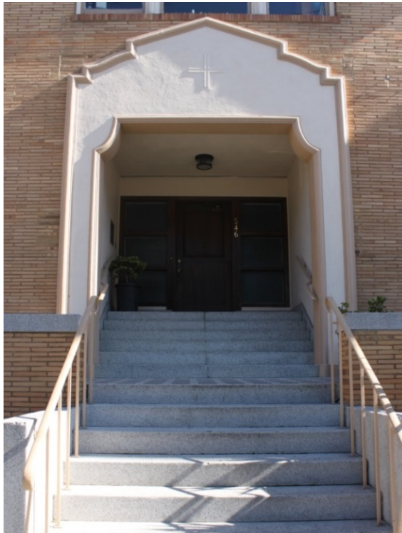
FIGURE 38 (LEFT). RECTORY: MAIN ENTRANCE, 2015.
