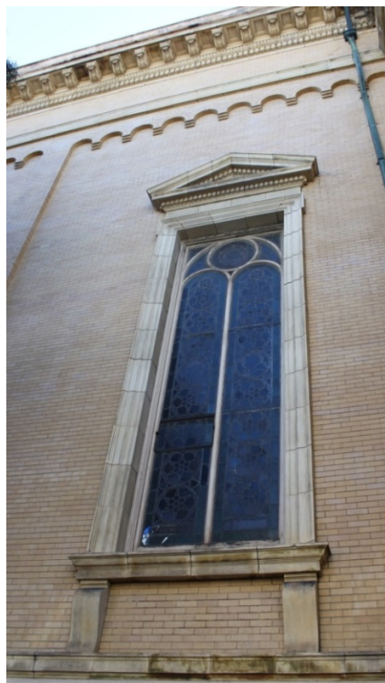
FIGURE 8. CHURCH: NORTH ELEVATION, DETAIL OF WINDOW, LOMBARDY BAND, AND CORNICE, 2015.
