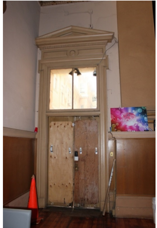
FIGURE 30: CHURCH: NAVE, SOUTH TRANSEPT ENTRY TO ALLEY, 2016.
