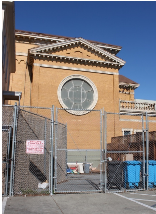
FIGURE 10: CHURCH: SOUTH TRANSEPT AND SACRISTY LOOKING NORTH FROM PARKING AREA OFF OAK ST., 2015.
