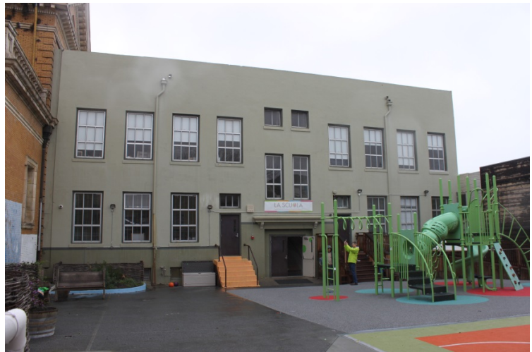
FIGURE 44. SCHOOL: REAR (SOUTH) ELEVATION AND SCHOOL YARD, 2016.
