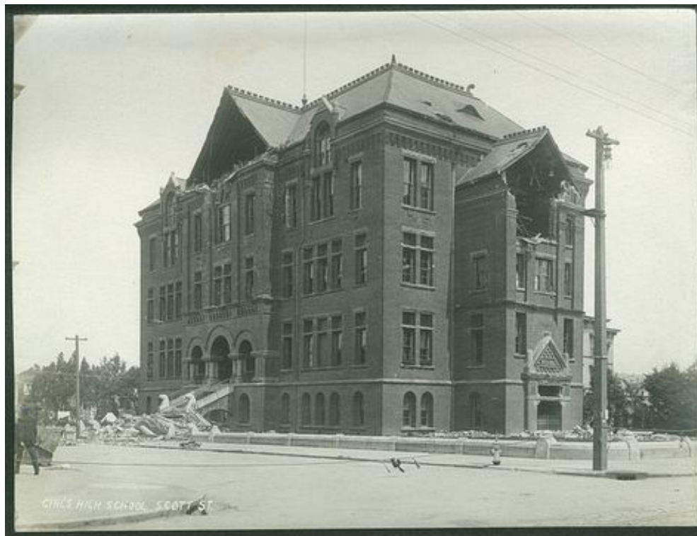
FIGURE 80. WELSH'S GIRLS HIGH SCHOOL AFTER DAMAGE IN THE 1906 EARTHQUAKE. SOURCE: DELGOYER LIBRARY, SOUTHERN METHODIST UNIVERSITY
