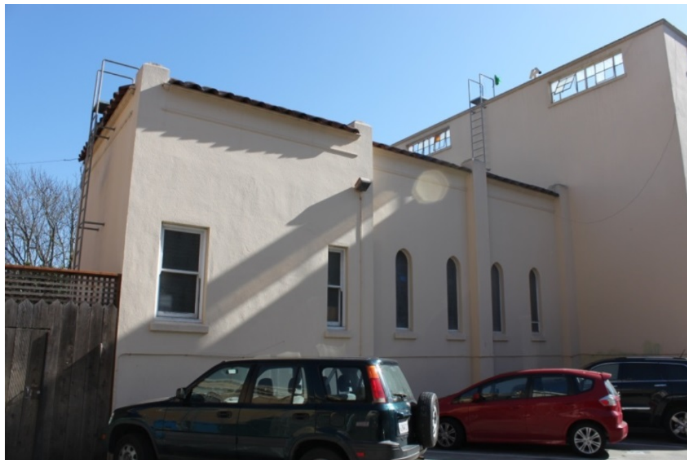
FIGURE 48. CONVENT, CHAPEL WING, LOOKING SOUTHEAST FROM PARKING AREA OF OAK ST., 2015.
