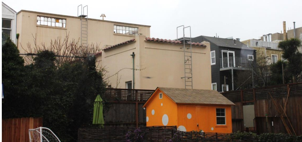
FIGURE 49. CONVENT: REAR (NORTH) ELEVATIONS OF CHAPEL ELL AND MAIN BLOCK, 2016.
