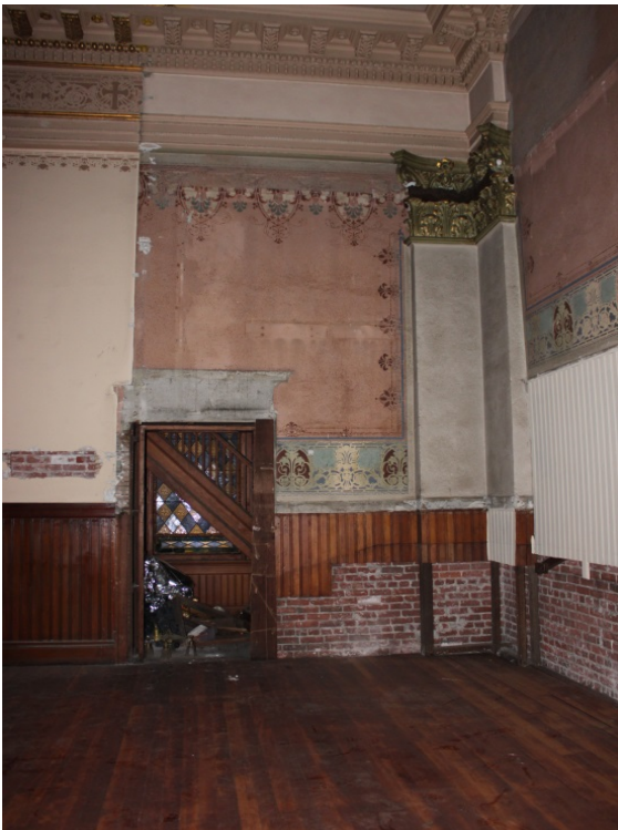
FIGURE 21. CHURCH: CHOIR LOFT, SOUTHWEST CORNER AND DOOR TO CONNECTOR TO RECTORY, 2016.
