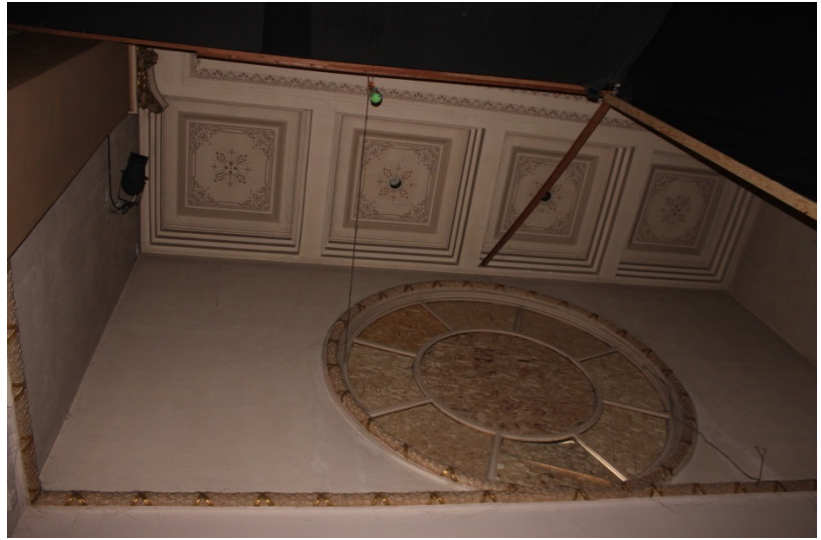
FIGURE 29: CHURCH: NORTH TRANSEPT SHOWING DECORATIVE DETAILING, 2016.
