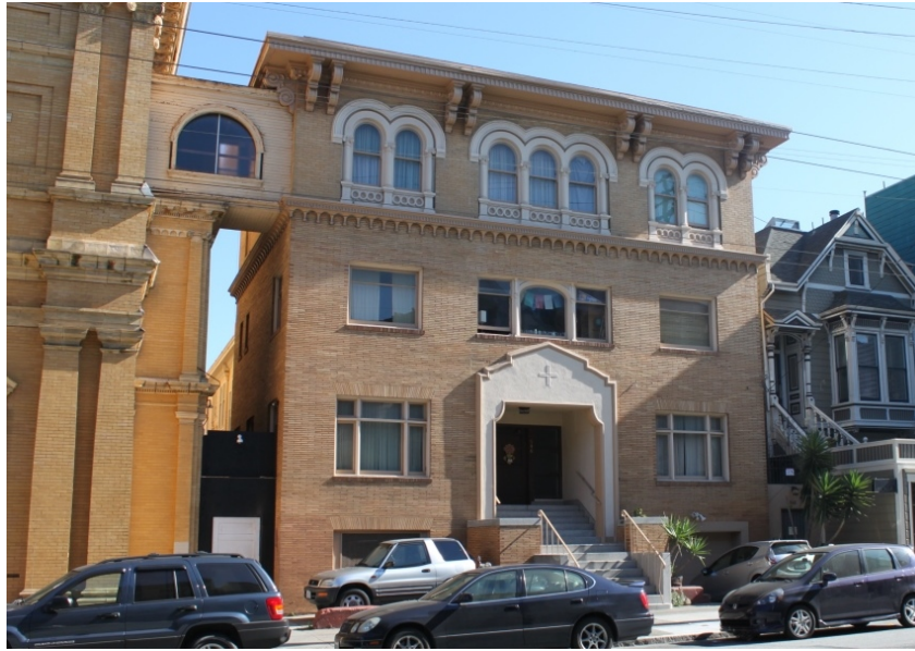
FIGURE 37. RECTORY: MAIN (WEST) ELEVATION FROM FILLMORE STREET, 2015.
