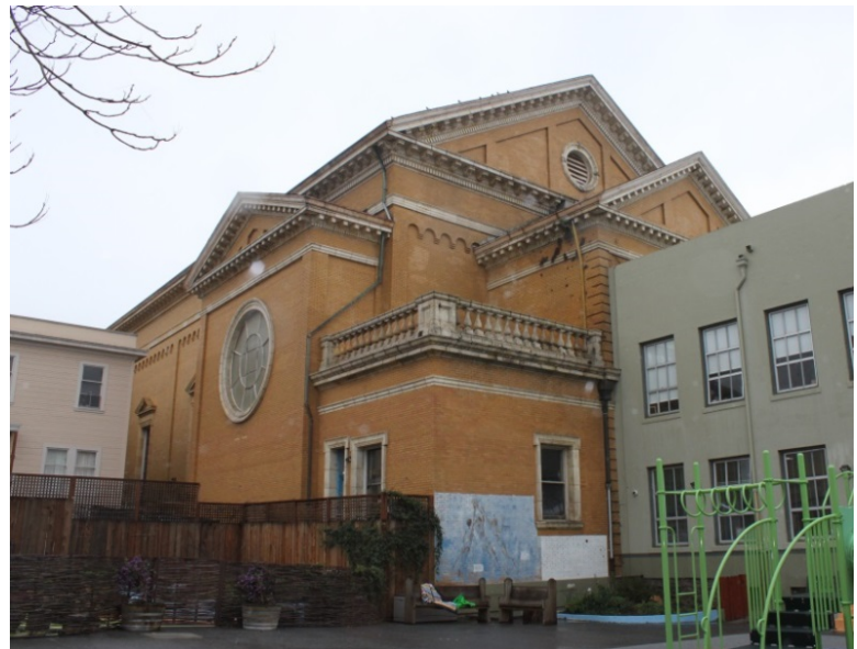
FIGURE 11. CHURCH: REAR, EAST ELEVATION FROM INTERIOR OF LOT, 2016.
