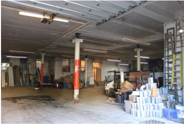
FIGURE 12. CHURCH: BASEMENT SHOWING GUTTED CONDITION, 2015.
