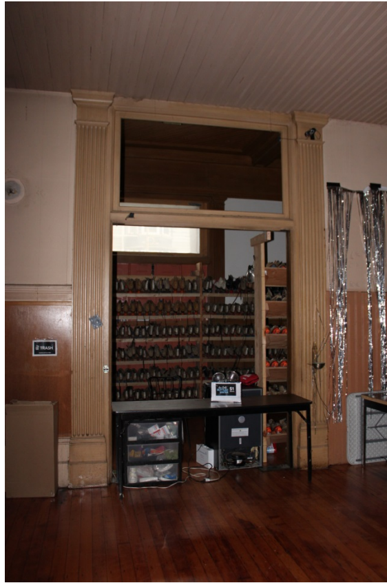
FIGURE 25. CHURCH: NAVE, NORTH DOOR FROM NARTHEX, 2016.
