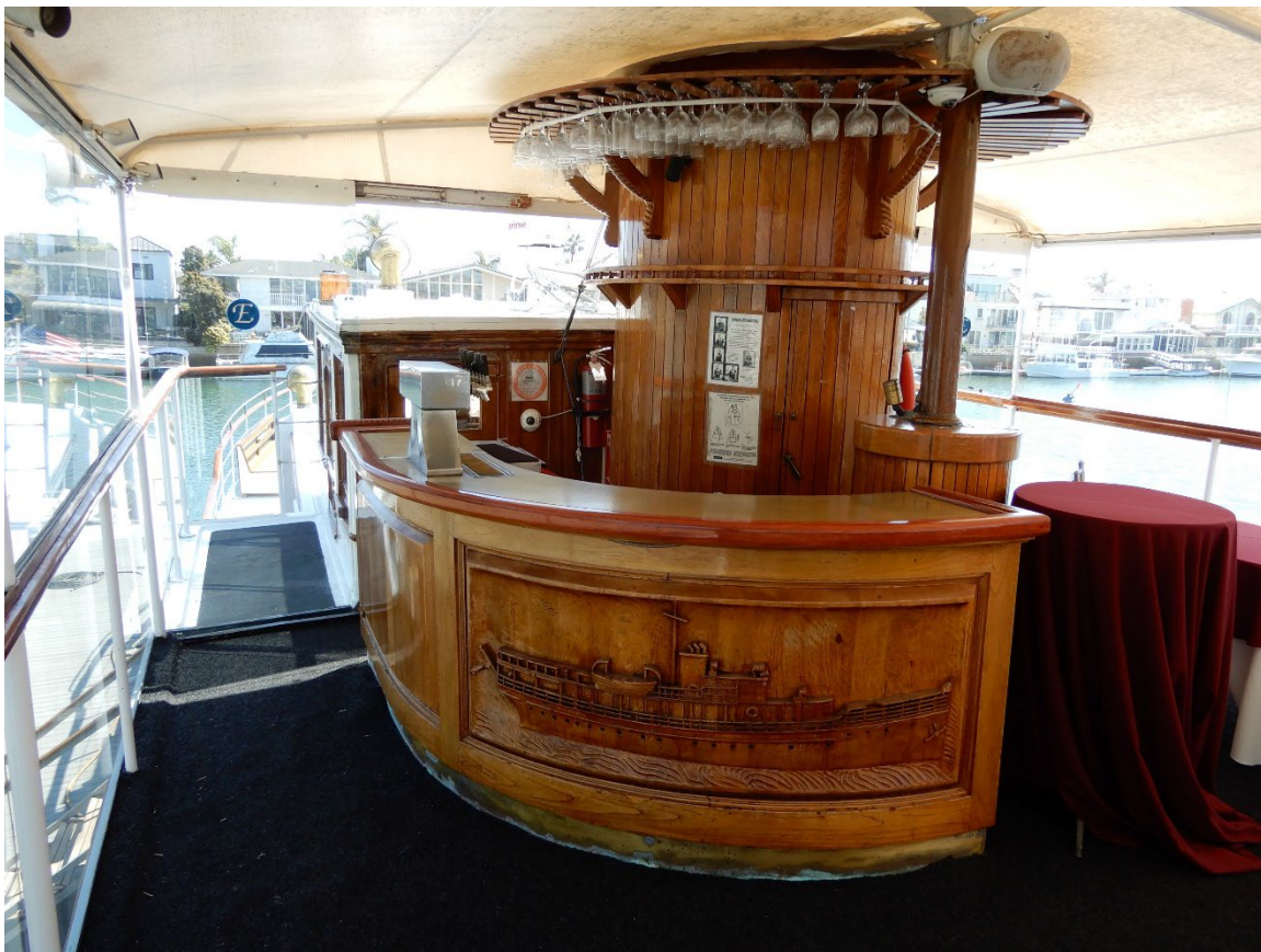
Figure 21. Upper deck, showing non-original teak bar with low relief portrait of Electra , and vertical teak paneling around the smokestack, designed and installed in 1994 (ARG, 2022)
