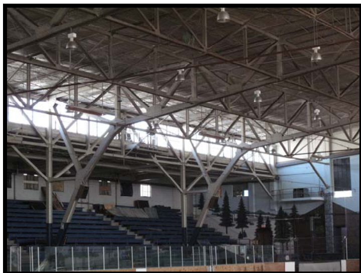
Photograph 10. Berkeley Iceland, Berkeley, Alameda County, California
