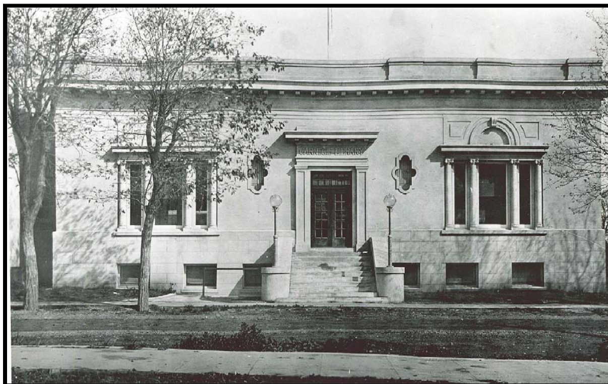
Photograph 44. Dixon Carnegie Library, Dixon, Solano County, California
