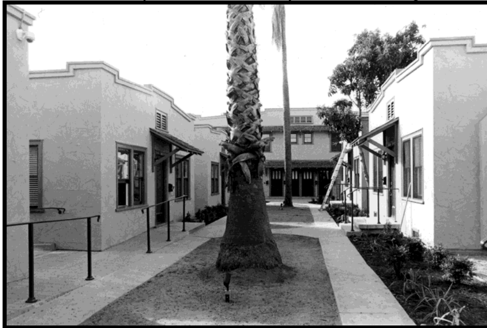
Photograph 19. 1721 North Kingsley Drive, Los Angeles, Los Angeles County, California
