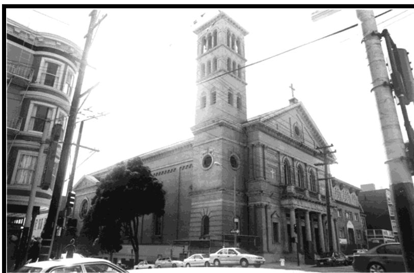
Photograph 36. Sacred Heart Church, San Francisco, San Francisco County, California
