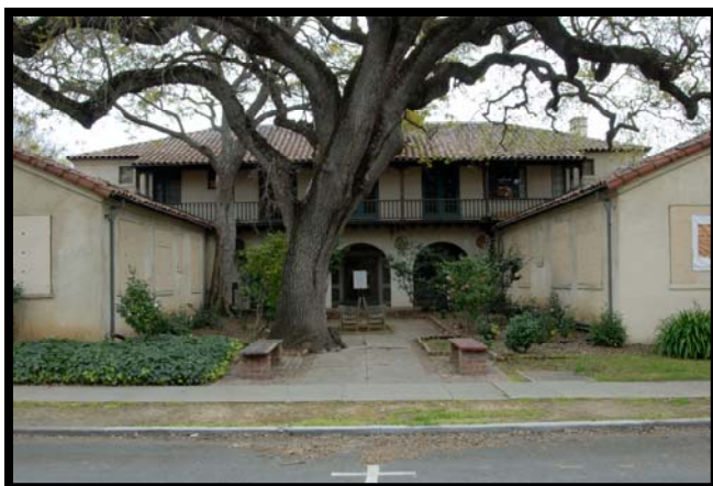
Photograph 42. Palo Alto Medical Clinic, Palo Alto, Santa Clara County, California
