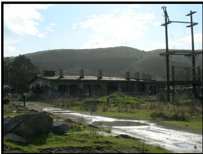
Photograph 41. Southern Pacific Bayshore Roundhouse, Brisbane, San Mateo County, California
