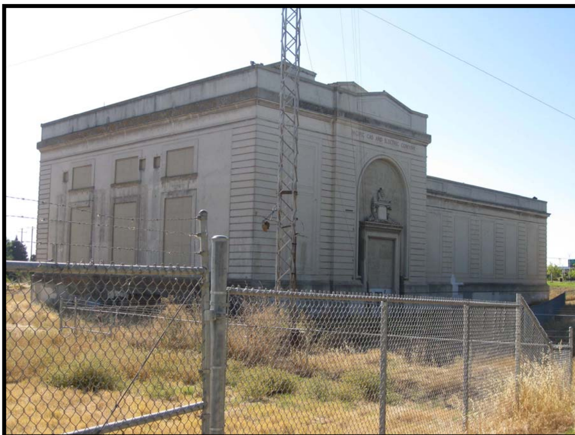
Photograph 32. PG&E Powerhouse, Sacramento, Sacramento County, California
