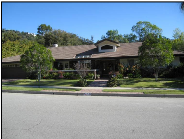
Typical residence from Pegfair Estates Historic District, Pasadena
