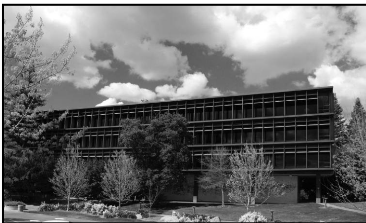
SMUD Building, Sacramento
