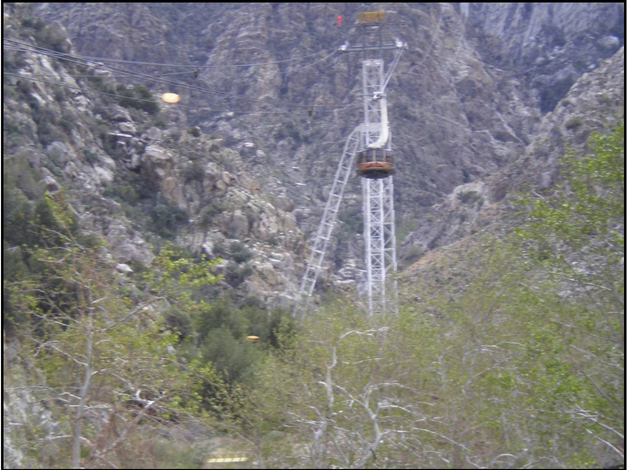
Commissioners ride the Palm Springs Tramway to Mount San Jacinto State Park.
