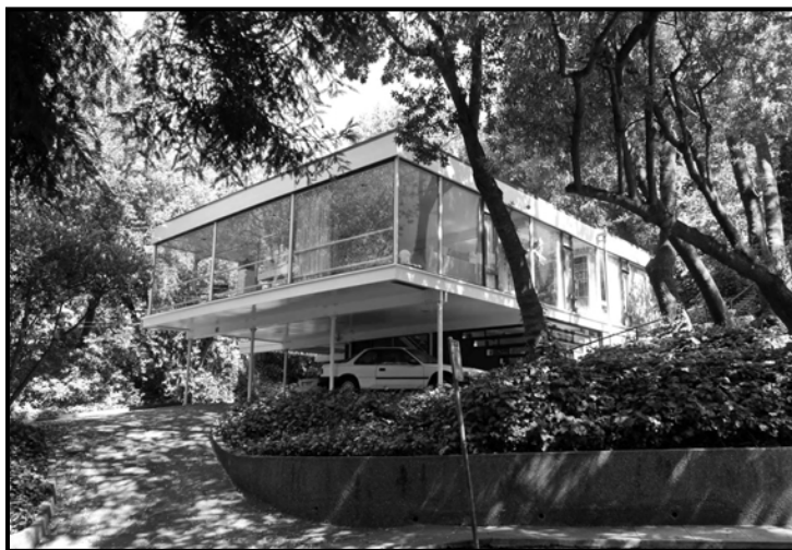
Olsen House, Berkeley
