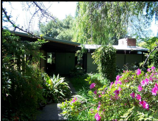
Photograph 22. Mello House, Pasadena, Los Angeles County, California
