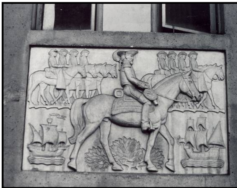
Photograph 30. Relief Detail of the Monterey County Courthouse
