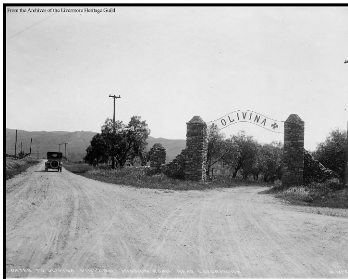
Photograph 46. Olivina Gate and Winery Ruins, Alameda County, California
