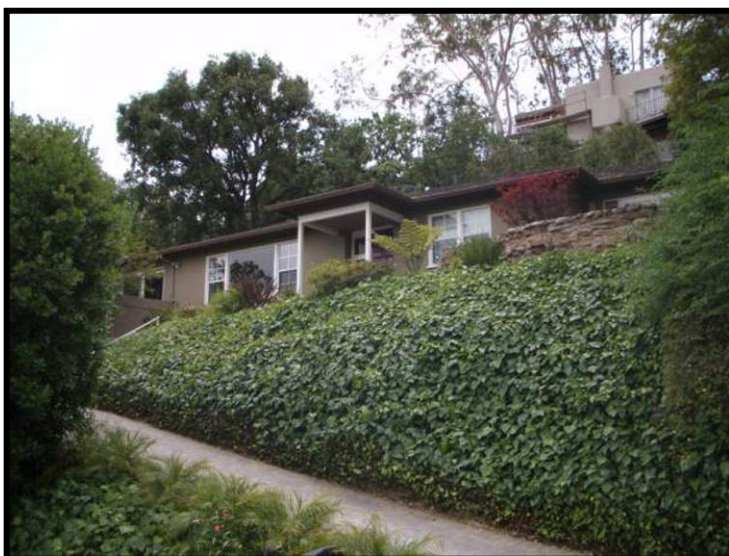
Photograph 26. Representative contributing resource in the Poppy Peak Historic District, Pasadena, Los Angeles County, California
