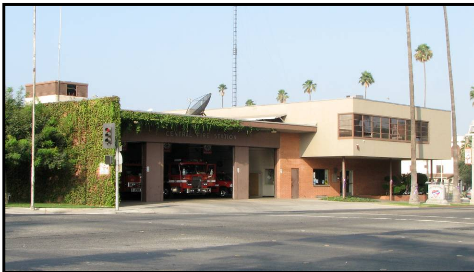
Photograph 45. Central Fire Station, Riverside, Riverside County, California
