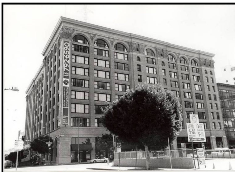
Photograph 18. Pacific Electric Building, Los Angeles, Los Angeles County, California
