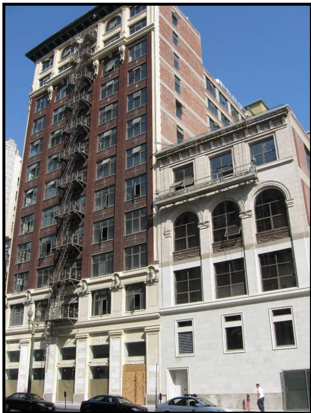
Photograph 27. Brockman Building and New York Cloak and Suit House (Annex), Los Angeles, Los Angeles County, California
