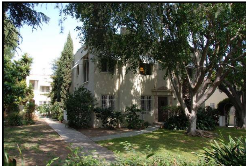
Photograph 16. Apartments at 1342-1346 N. Hayworth Ave., West Hollywood, Los Angeles County, California
