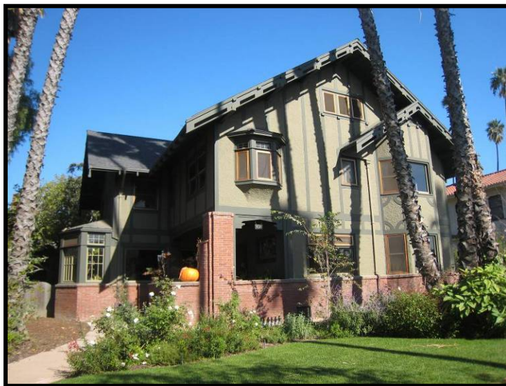
Photograph 15. The Holmes-Shannon House, Los Angeles, Los Angeles County, California
