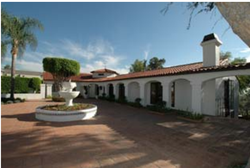
Photograph 44. Edson House, Orange County, California
