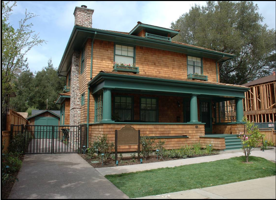
Hewlett-Packard House and Garage, Palo Alto, Santa Clara County. Listed on the National Register of Historic Places April 20, 2007 at the national level of significance.
