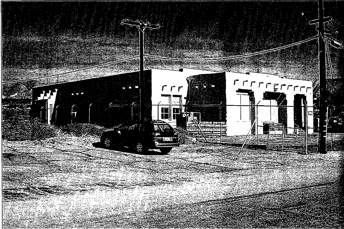
ATTRepeater2. South-facing primary façade and west-facing elevation; view toward the northeast.
