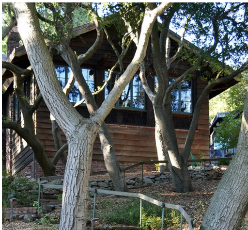
Cottage in North Berkeley with rustic qualities of the First Bay Tradition and Simple Home principles, 1915.
