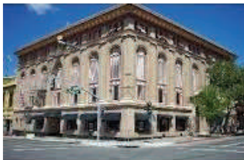
Vallejo used CDBG funds to adaptively reuse its masonic temple as a live-work project
