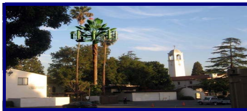
Photo Simulation of a Monopalm Installation St. Elizabeth of Hungary Catholic Church Altadena, California
