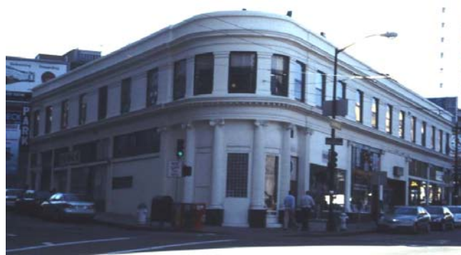
Colombo Building, San Francisco City and County, listed January 31, 2008
