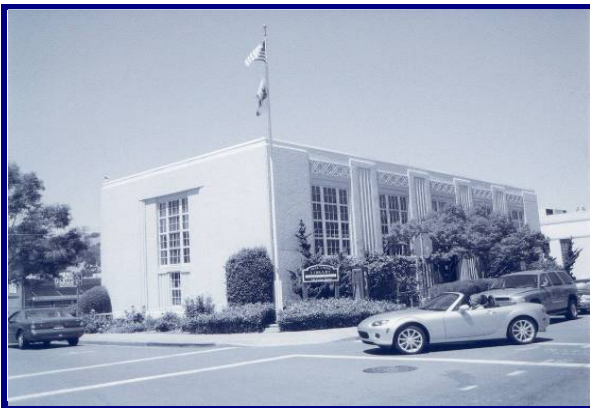
Martinez City Library, Martinez, Contra Costa County, listed January 31, 2008
