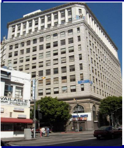
Board of Trade Building, Los Angeles, Los Angeles County, listed January 24, 2008
