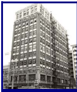
Garment Capitol Building Los Angeles, Los Angeles County Listed March 8, 2010
