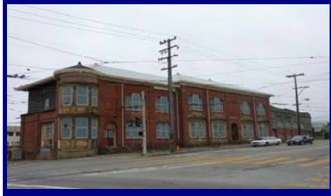
Geneva Office Building & Powerhouse San Francisco, San Francisco County Listed March 31, 2010
