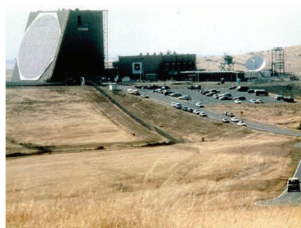
PAVE PAWS Installation, Beale AFB
