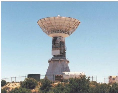
La Posta Radar Installation
