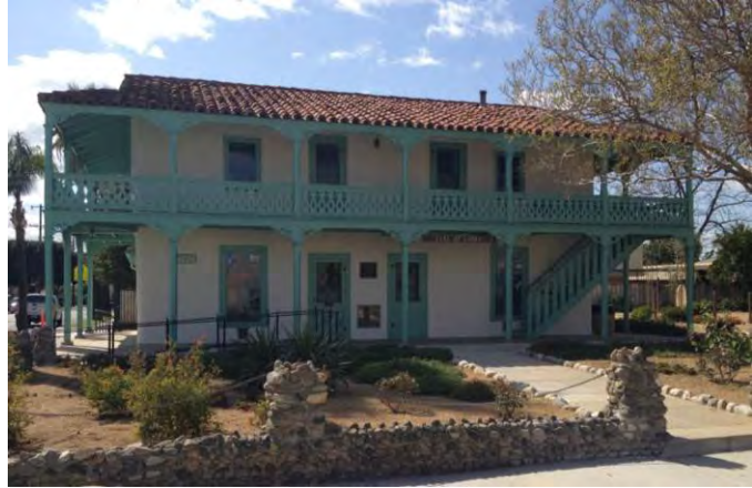
The Lopez Adobe in San Fernando was one of the many historic buildings damaged in the 1994 Northridge Earthquake.
