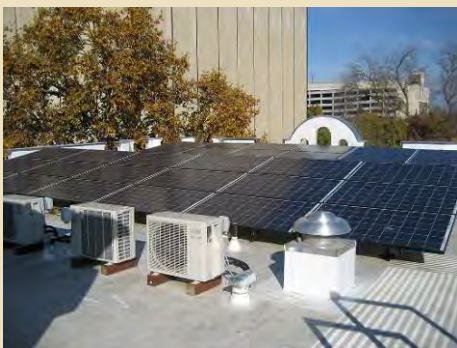
Low-profile photoelectric panels on the roof helped the building achieve LEED silver certification.
