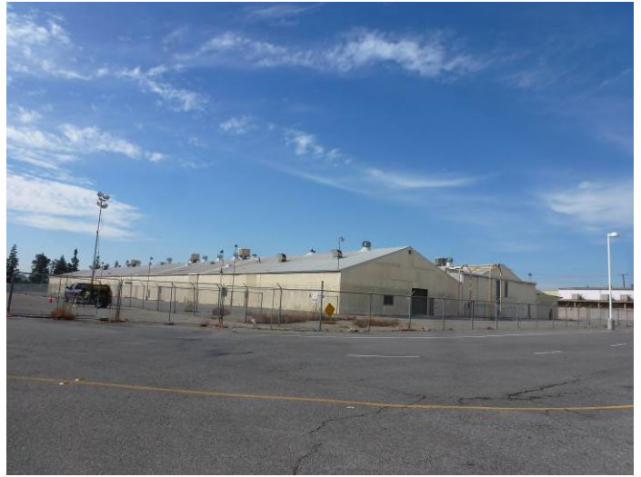
Image 2. View looking west at the northeast and southeast façades.
