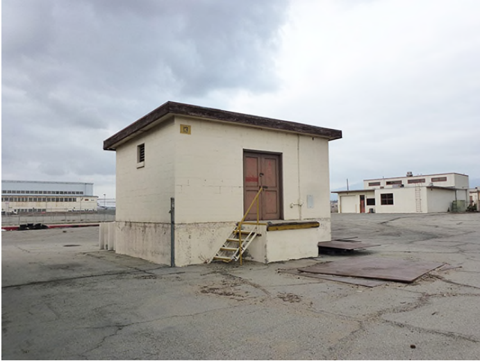
Image 1. View looking northwest at the south and east façades.
