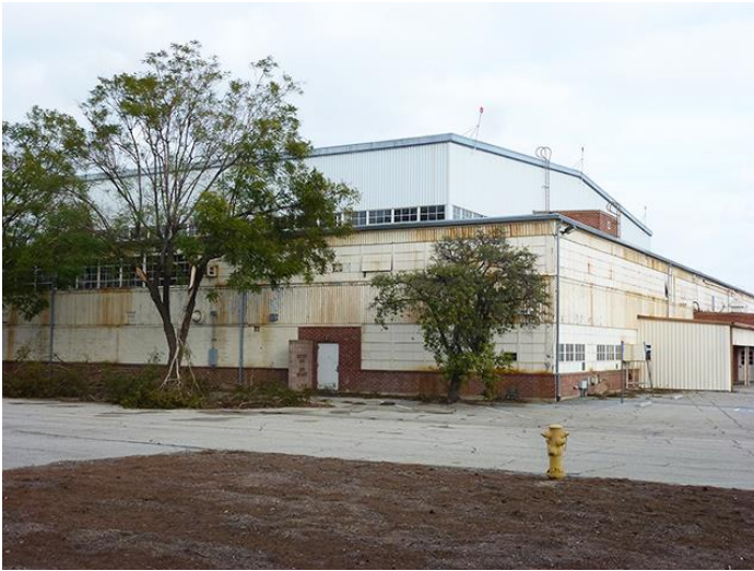
Image 5. Looking southwest at the north and east façades.
