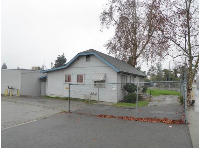
Image 1. View looking southwest at the east and north façades.
