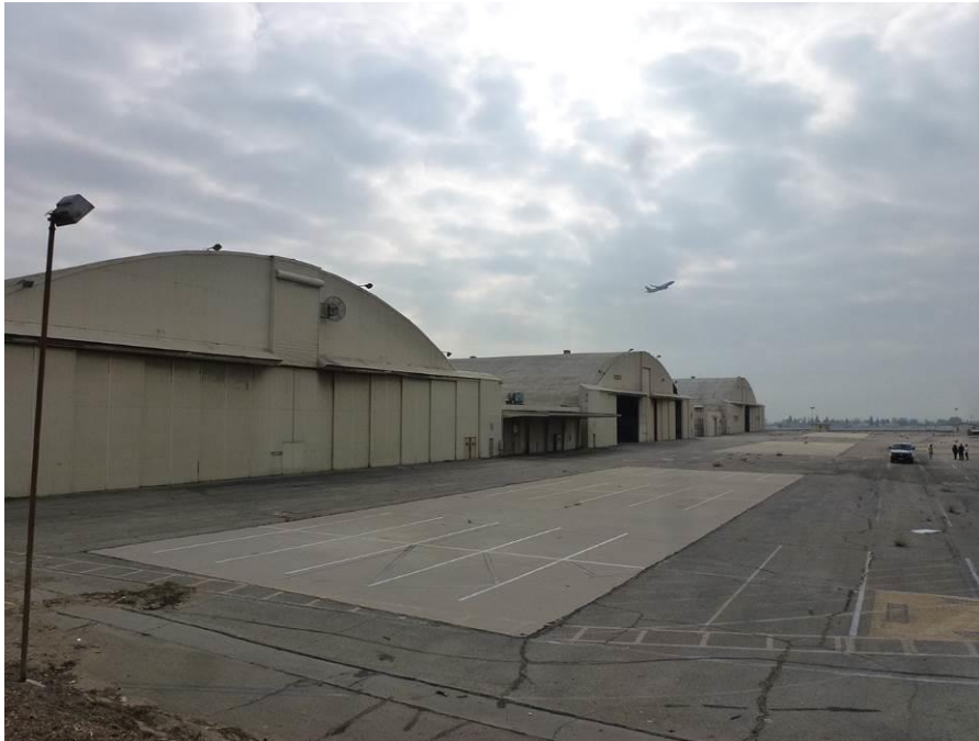
Image 3. View looking southeast at the west and north façades of hangars 6, 4, and 2.
