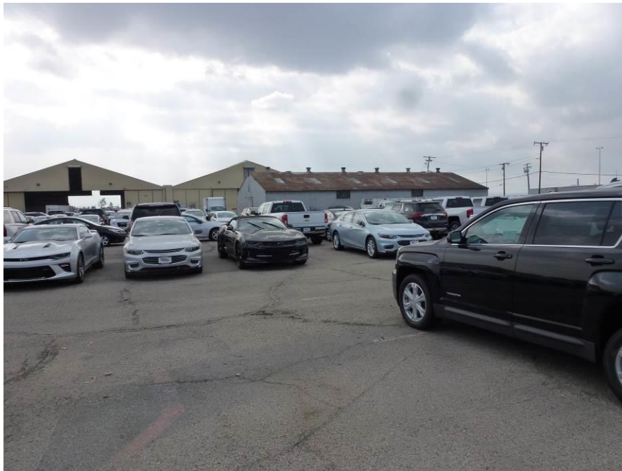
Image 6. View looking southwest at the east and north façades of Building 21.
