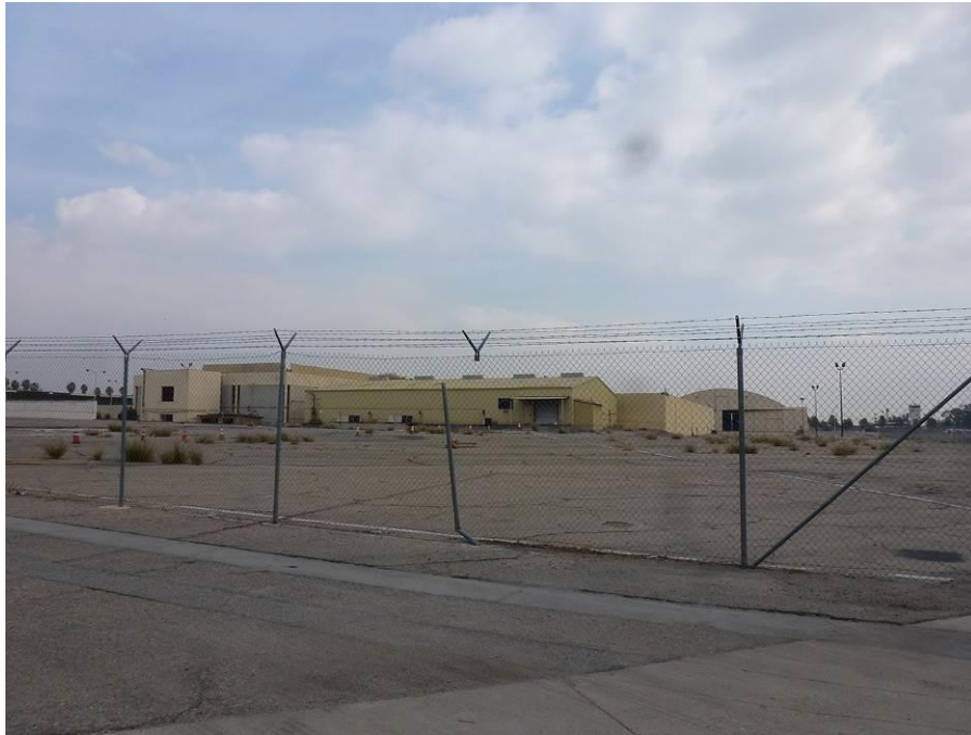
Image 5. View looking northwest at the LAS facilities.
