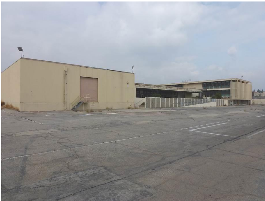
Image 2. View looking northwest at the east façades of the Mail Room, the Cafeteria, and the Executive Office Building.
