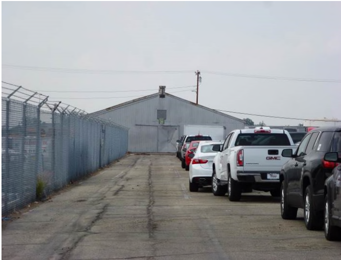
Image 1. View looking west at the east façade.
