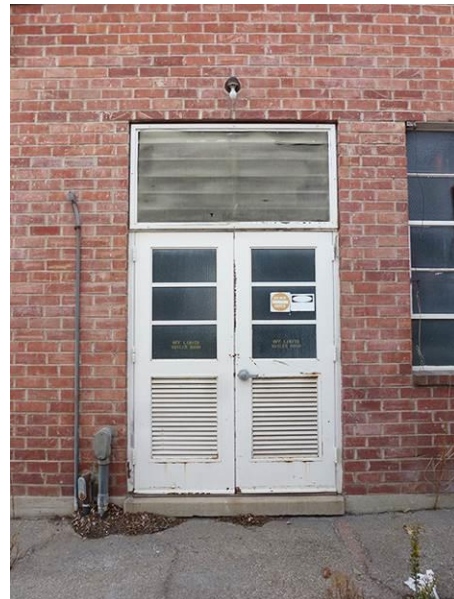
Image 8. Detail view of the entrance on the east façade of the Diesel Tanks room.
