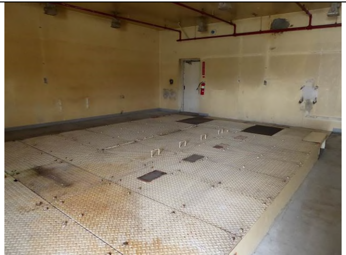
Image 8. Detail view of the interior looking west.
