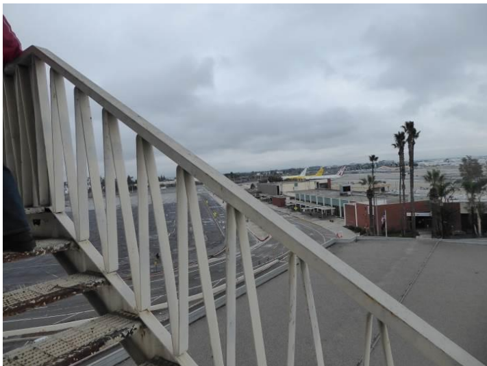
Image 7. View from the exterior staircase looking toward Terminal One from the Control Tower.
