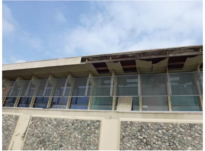
Image 6. Detail view of the south façade.
