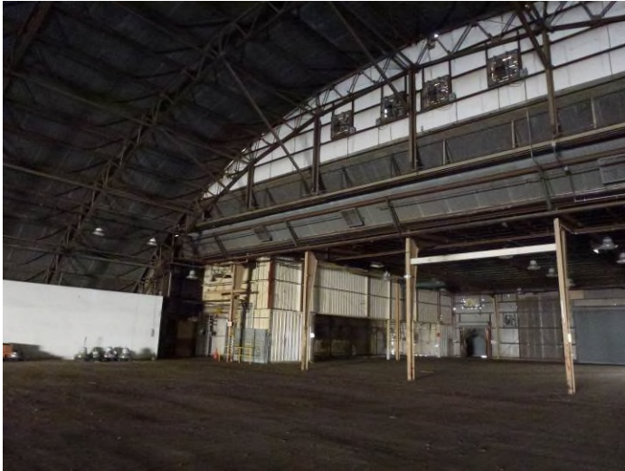
Image 5. Detail interior view looking east.
