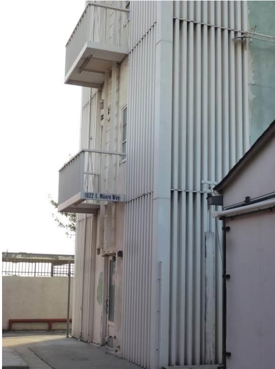
Image 9. Detail view of the primary entrance on the east façade.
