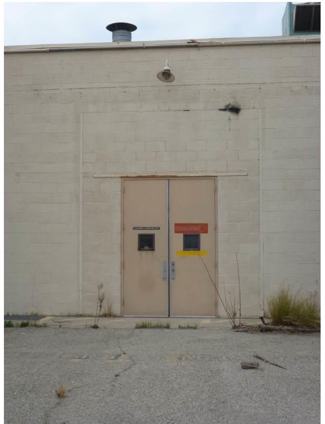
Image 2. Detail view looking west at the east façade.
