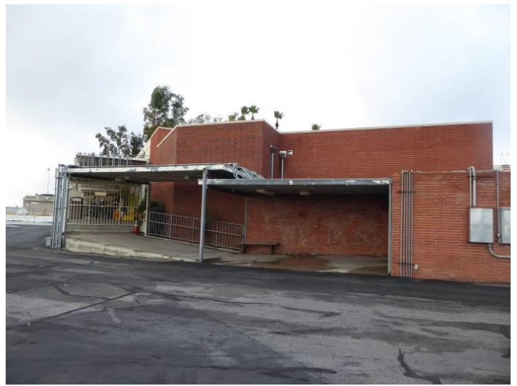
Image 20. View looking northwest at the south façade of the USO building (formerly the West Lobby).
