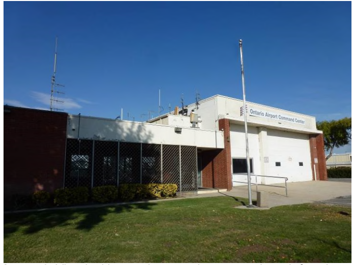
Image 2. View looking northeast at the west and south façades.
