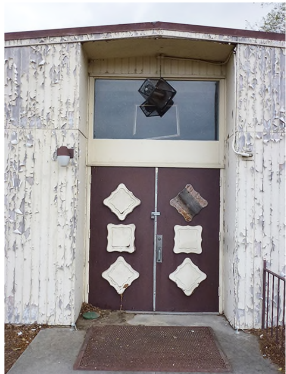
Image 4. Detail view of the primary entrance at the north façade.
