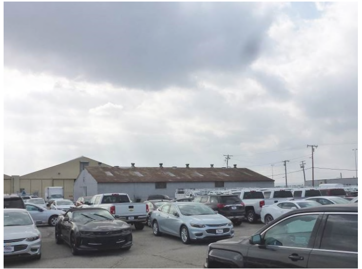
Image 4. View looking southwest at the north and east façades.
