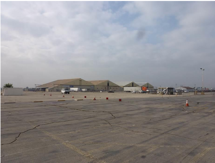
Image 4. View looking southwest and the east and north façades of hangars 20 and 19.
