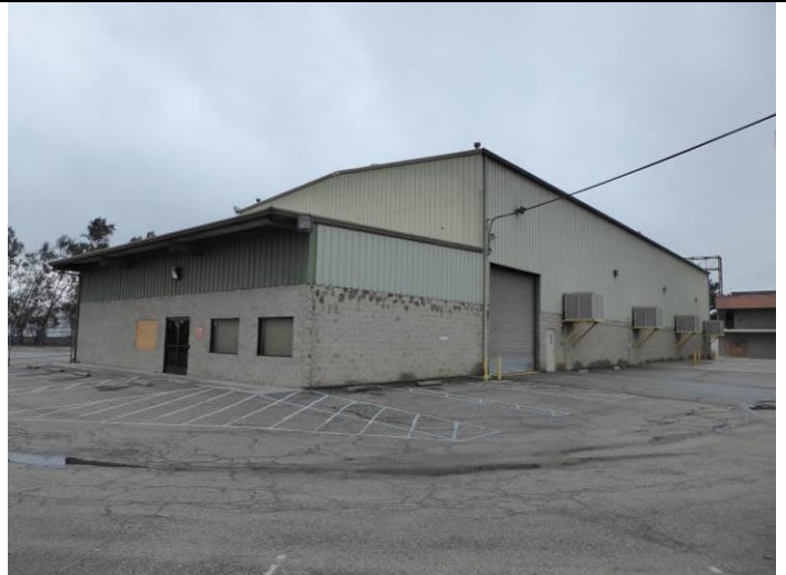
Image 16. View looking southwest at the north and east façades of the Prep-to-Test building and offices.
