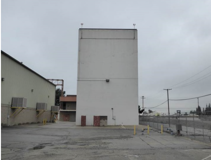
Image 13. View looking west of the east façade of Test Cell 2.
