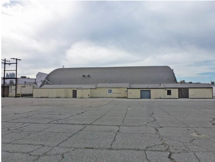
Image 3. View looking southwest at the northeast façade of ancillary buildings M, with Hangar 4 in the background. ASM, December 1, 2016.
