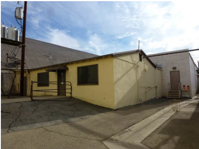
Image 11. View looking east at the northwest and southwest façades of Building 21.
