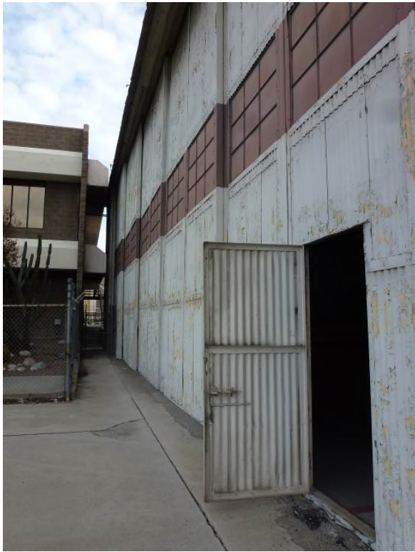
Image 3. Detail view looking at the northwest façade.
