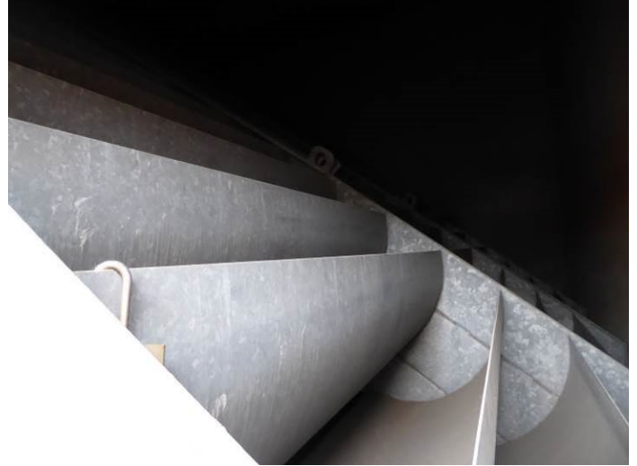
Image 6. Detail view of intake vents in interior at west end.
