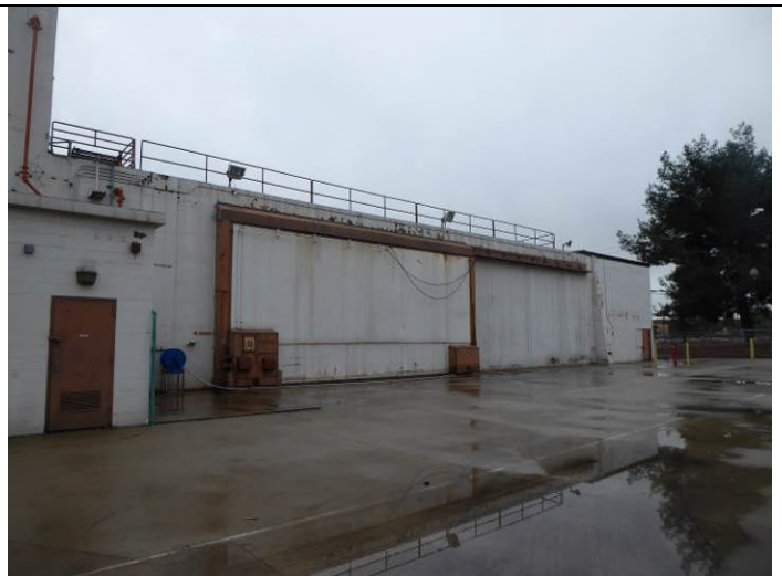
Image 4. Detail view looking southwest at the north façade of Test Cell 1.
