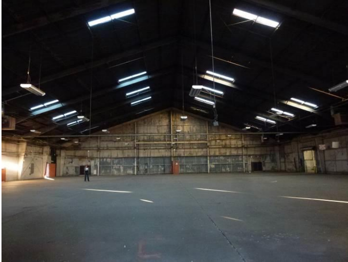
Image 5. Interior view looking southwest.
