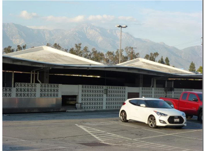
Image 6. Detail view looking north at the southwest façade of Baggage Claim B. This building is recommended as a contributor to the historic district.
