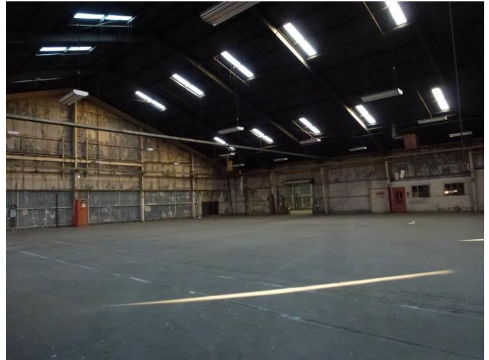
Image 4. Interior view looking southeast.
