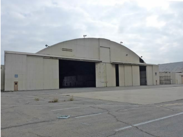
Image 1. View looking southeast at the west façade.
