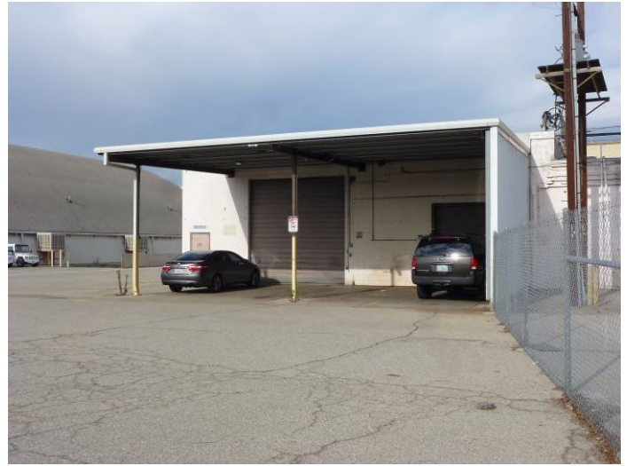
Image 6. View looking west at the southeast and northeast façades of Building G.
