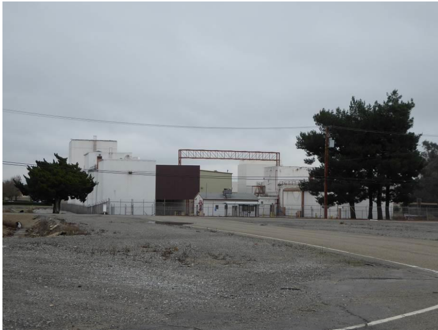
Image 6. Detail view looking south at the north façade of Test Cell 1. ASM, December 1, 2016.
