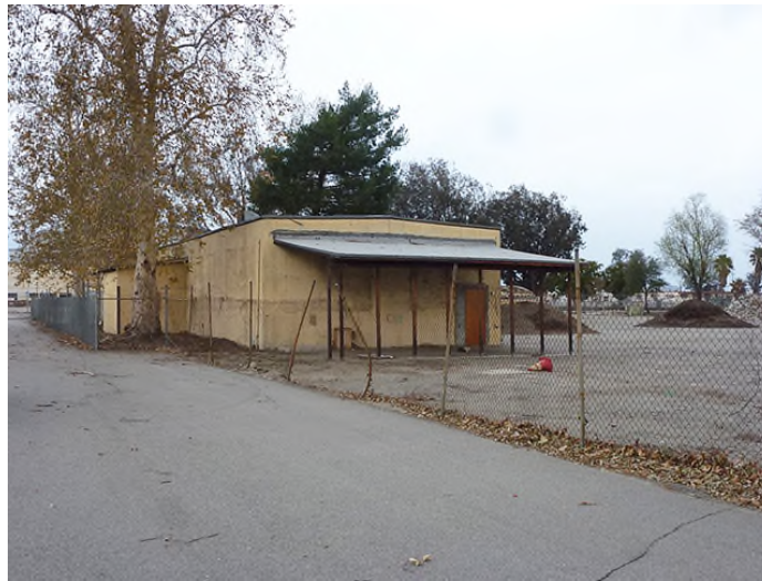
Image 3. View looking northeast at the west and south façades.
