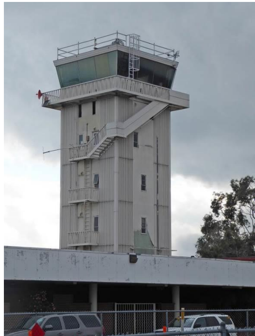
Image 7. View looking southwest at the east and north façades of the Control Tower. The Control Tower is recommended as a contributor to the historic district.
