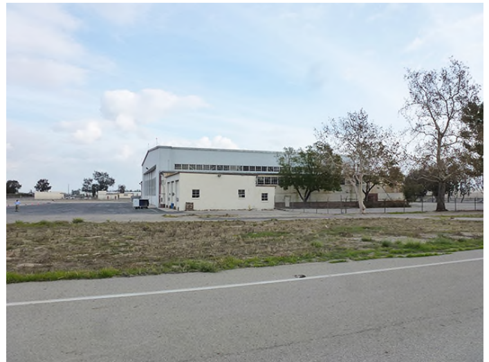
Image 2. View looking east at the west façade.
