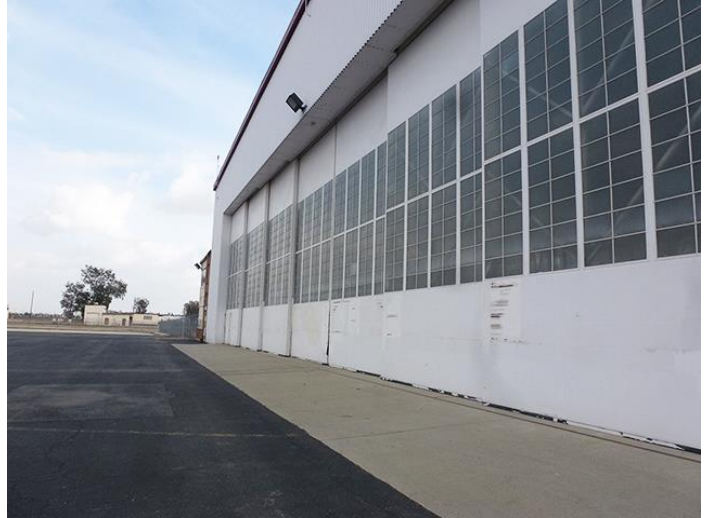
Image 2. View looking east at the west façade.
