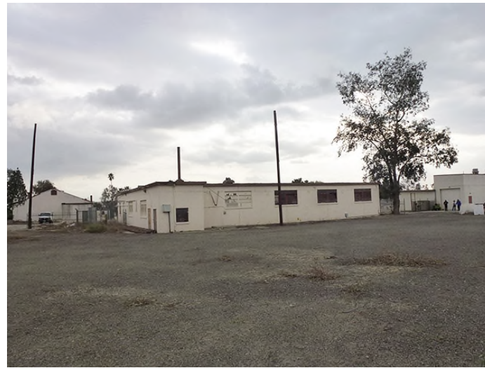
Image 3. View looking southwest at the east and north façades.
