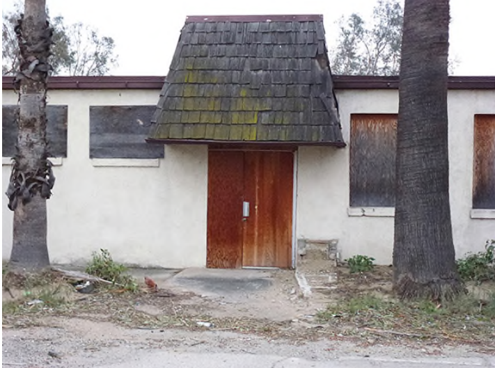
Image 1. Detail view of the primary entrance at the north façade.
