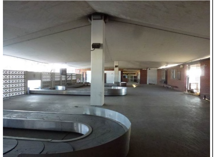
Image 4. Interior view looking west.
