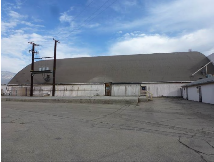
Image 1. View looking northeast at the southwest façade.
