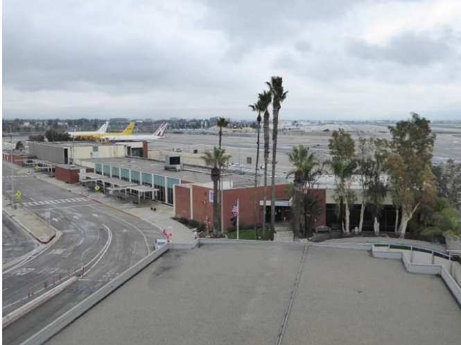
Image 1. View of Terminal One and ancillary buildings looking east from the Control Tower cab.
