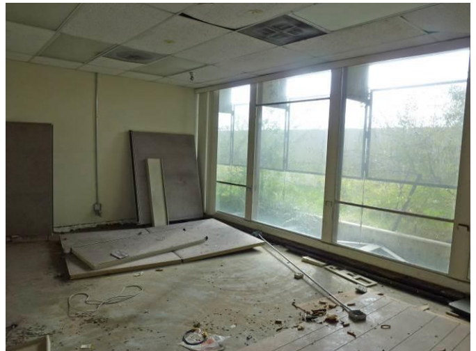
Image 8. View of the first-floor interior looking southeast.
