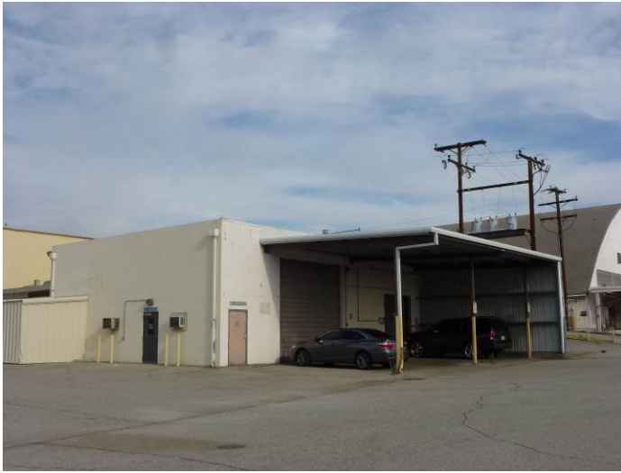
Image 5. View looking north at the southwest and southeast façades of Building G.
