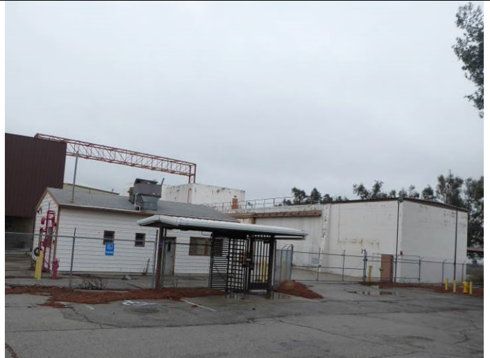
Image 2. View looking east at the northwest and southwest façades of the Guard House and Test Cell 1.
