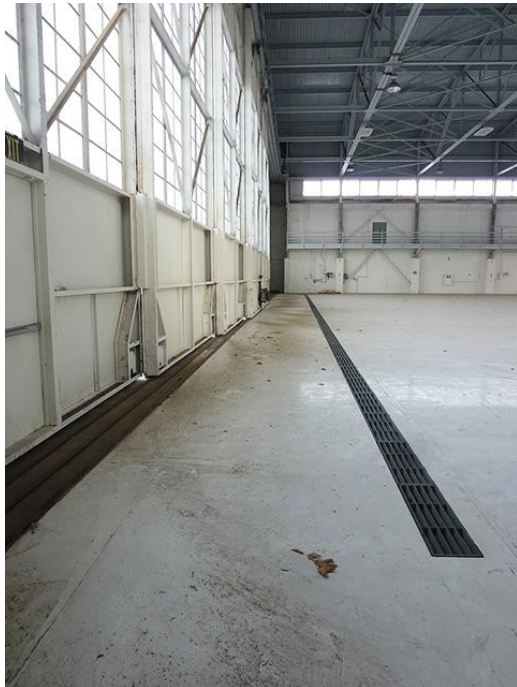
Image 15. Detail interior view of the hangar doors looking east.
