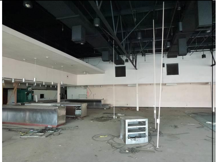
Image 4. Interior view looking southwest.
