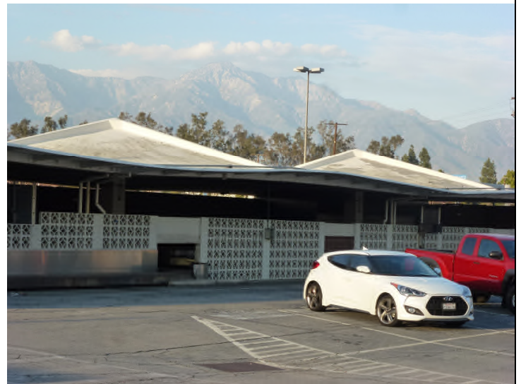
Image 2. Detail view looking north at the southwest façade.
