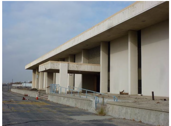
Image 4. Detail view looking northeast at the south façade.
