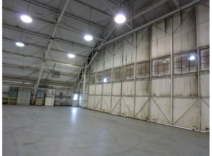
Image 6. Detail view of the interior looking west.
