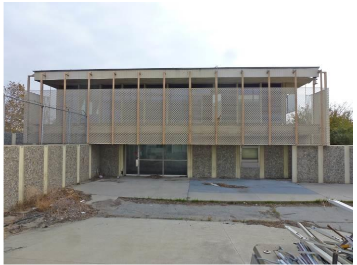
Image 2. View looking east at the west façade.
