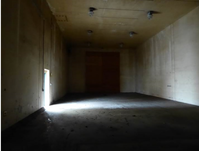
Image 9. Interior view of Test Cell 1 looking east.
