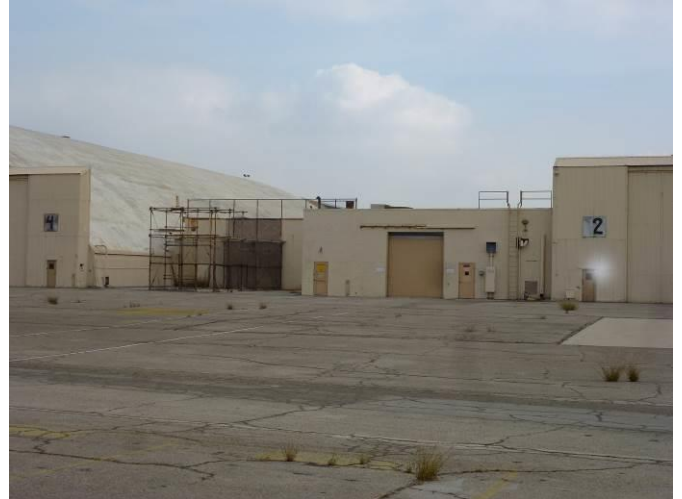
Image 2. View looking east at the west façade.
