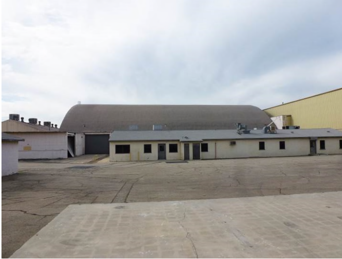
Image 1. View looking southwest at the northeast façades of Hangar 3 and the Commissary Building.
