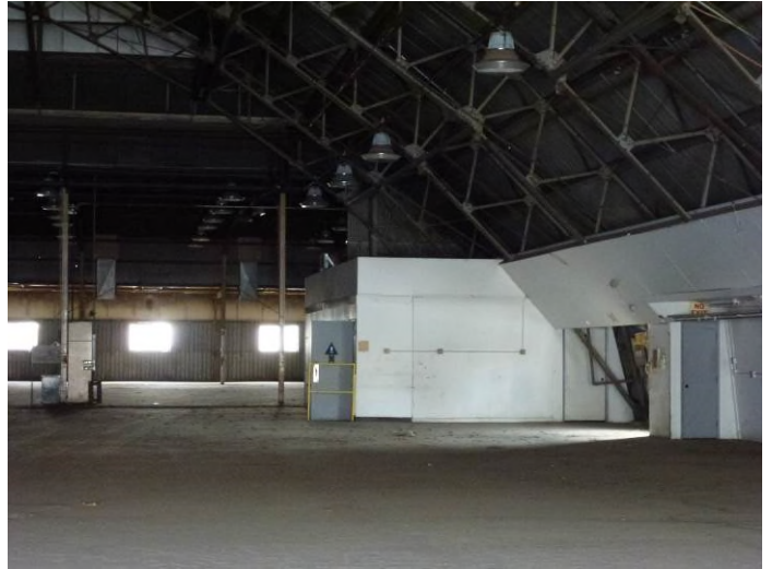
Image 6. Interior view looking southeast.
