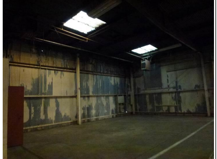
Image 6. Interior view of south wing.
