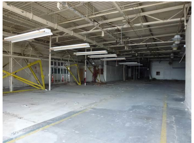
Image 4. View of the interior looking southwest.
