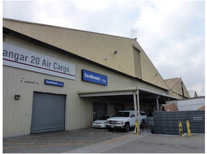
Image 2. Detail view looking southwest at the north façade.
