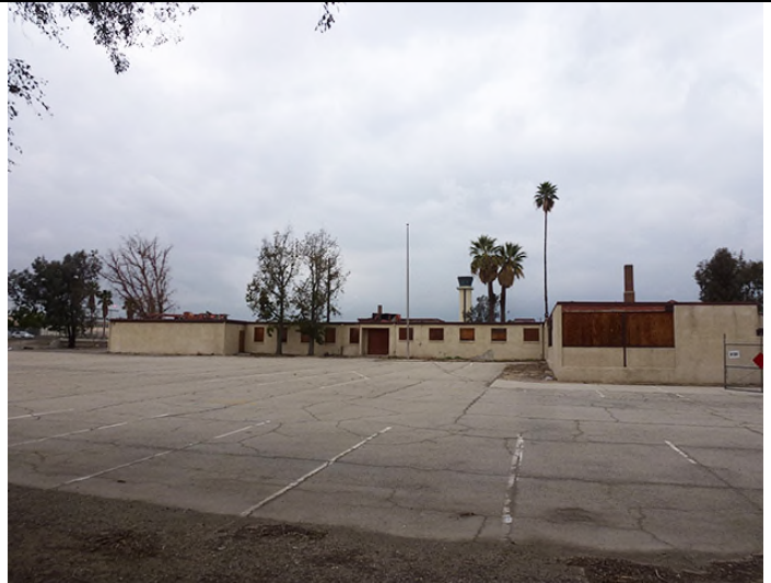
Image 4. View looking north at the south façade.
