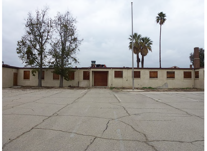
Image 6. Detail view of the south façade.
