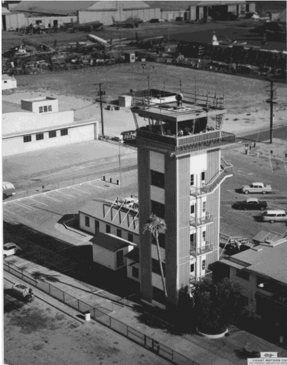
Image 13. View looking northwest at the south and east facades, ca. 1960. Source: Virgil R. Percy, photographer, July 18, 1969 [in Model Colony Room photo archives].
