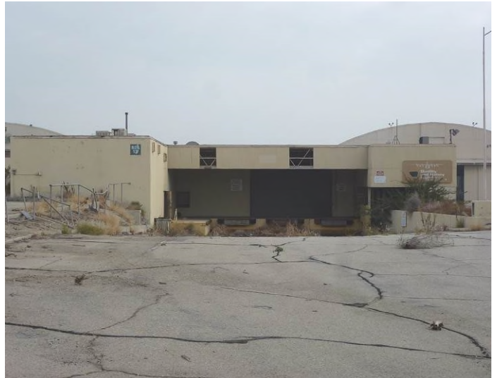
Image 2. View looking east at the west façade.
