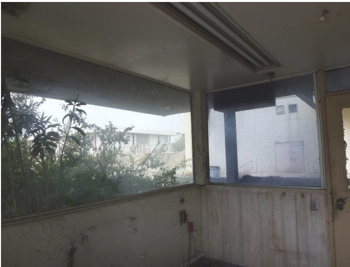
Image 3. From the interior looking northwest.
