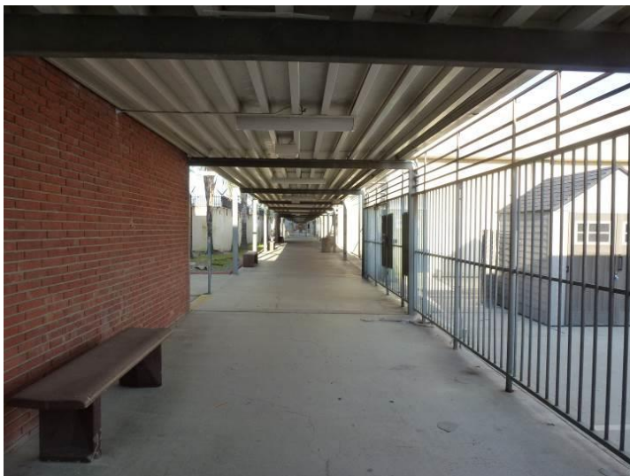
Image 15. View looking northeast at the passenger arcade behind Terminal One. As a later addition to the terminal, this portion of the building does not contribute to the historical significance.
