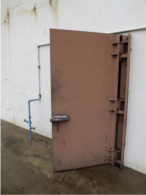
Image 5. Detail view of steel personnel door on north façade.
