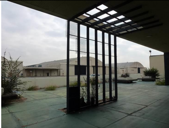
Image 3. Detail view looking southeast from Building 11.
