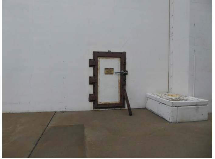
Image 14. Detail view looking north at the south façade of Test Cell 2.
