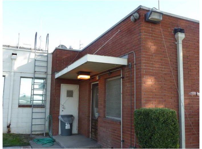
Image 10. Detail view looking southeast at the north entrance to the personnel quarters.
