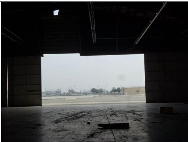
Image 5. View from the interior looking east.
