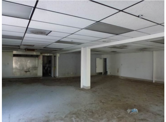
Image 10. Interior view of the Commissary Building.
