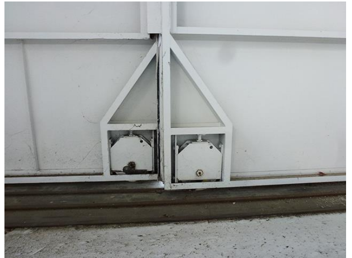
Image 16. Detail view of the hangar door track mechanism.
