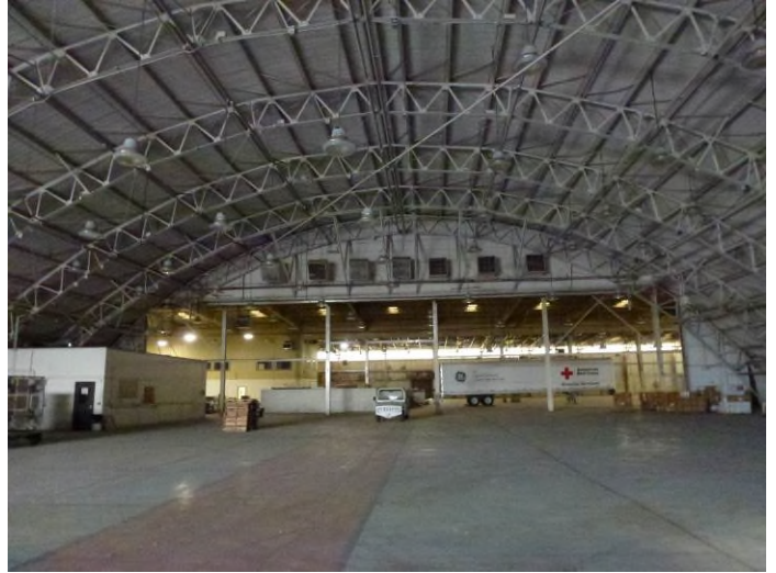
Image 2. Interior view looking northwest.
