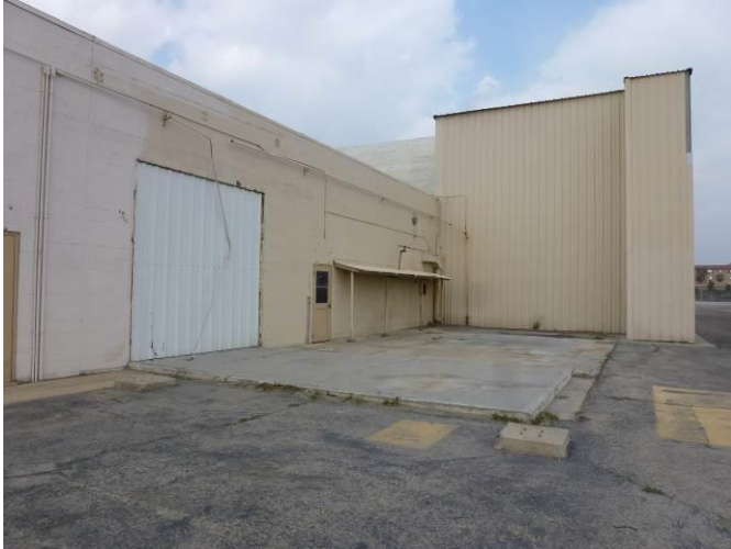
Image 1. View looking northwest at the east façade, with the south façade of Hangar 2 to the right.
