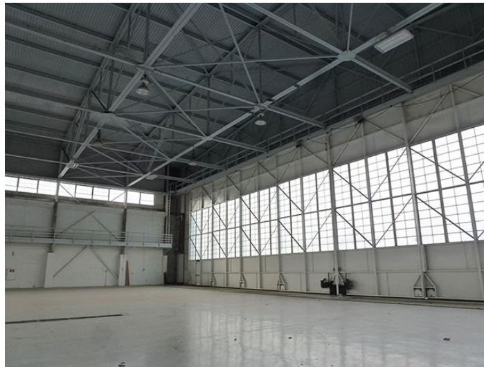
Image 11. Interior view of the hangar looking northwest.
