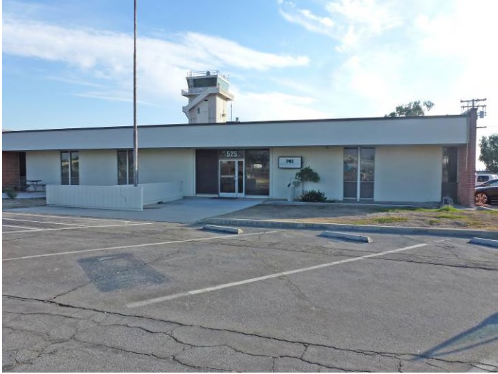
Image 1. View looking south at the north façade.
