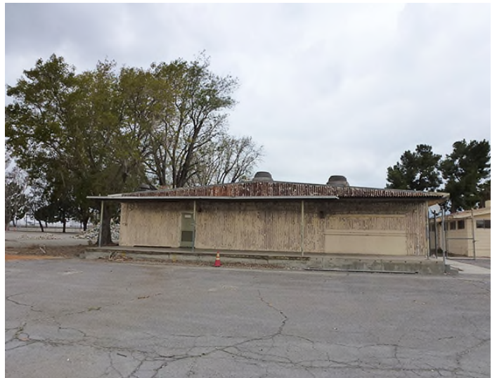
Image 2. View looking north at the south façade.
