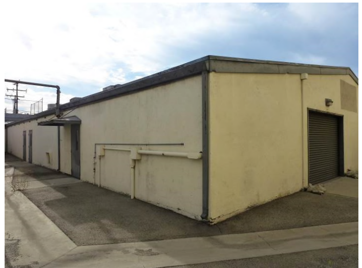
Image 2. View looking south at the northeast and northwest façades of Building E.
