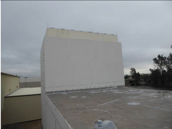
Image 1. View looking north at the southeast and northeast façades of Test Cell 1.
