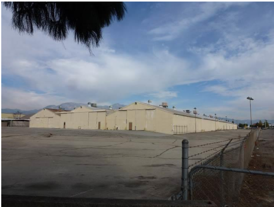
Image 4. View looking north at the southwest and southeast façades of the Storage Hangars. ASM, December 1, 2016.
