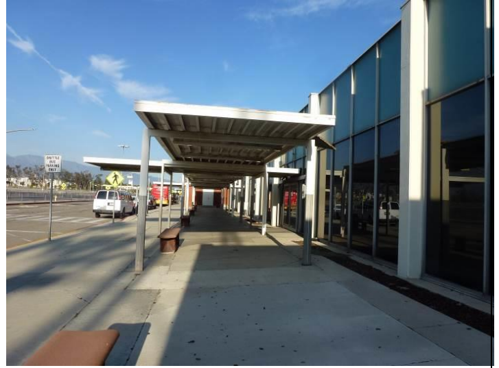
Image 2. Detail view looking northeast at the northwest façade.
