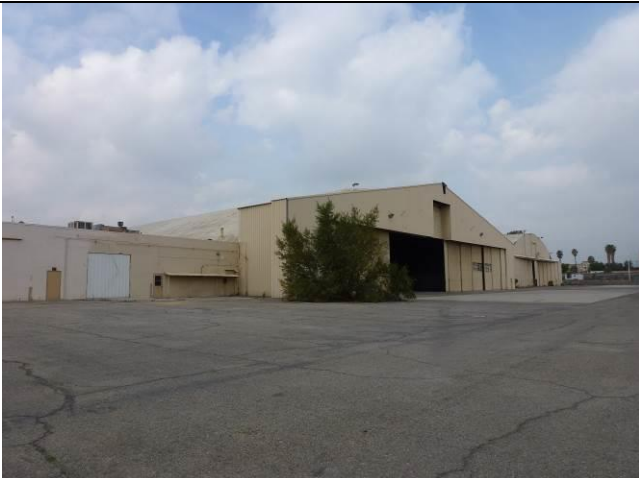
Image 3. View looking northwest at the east façade.
