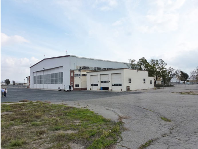
Image 1. View looking southeast at the north and west façades, with the hangar in the background.
