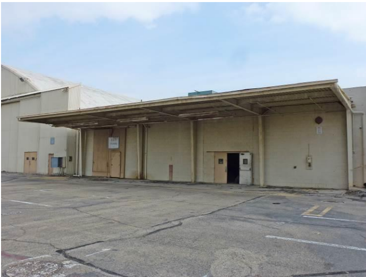
Image 1. View looking northeast at the west façade.
