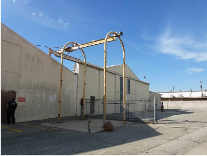
Image 5. View looking west at the northeast façade.
