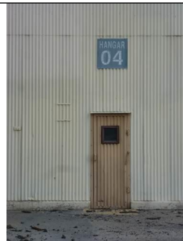
Image 6. Detail view looking east at west façade.
