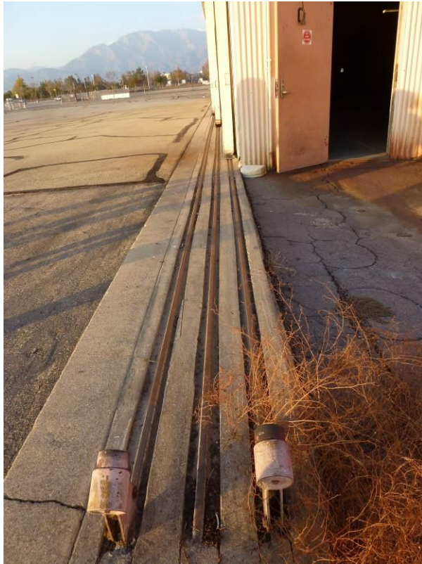
Image 3. Detail view looking north at the rails on the west façade.
