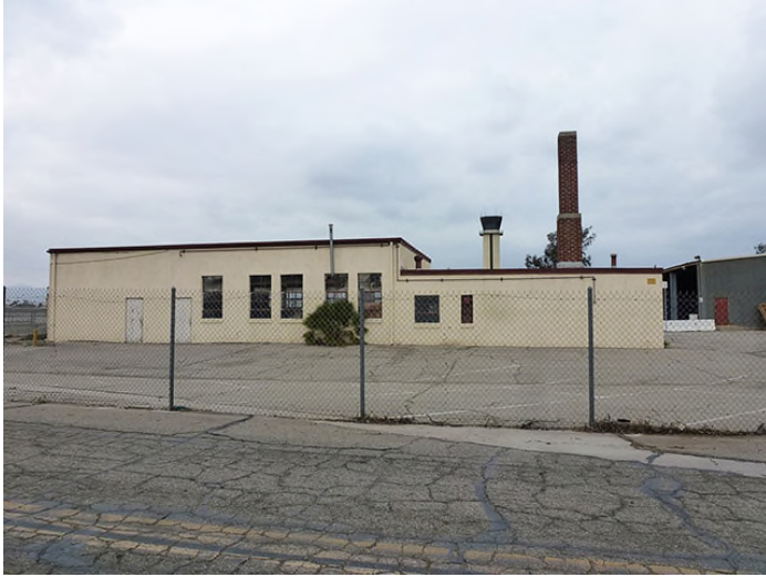
Image 1. View looking north at the south façade.
