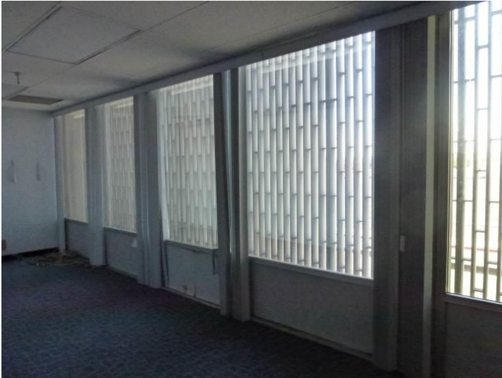
Image 9. Interior view of second-floor offices.
