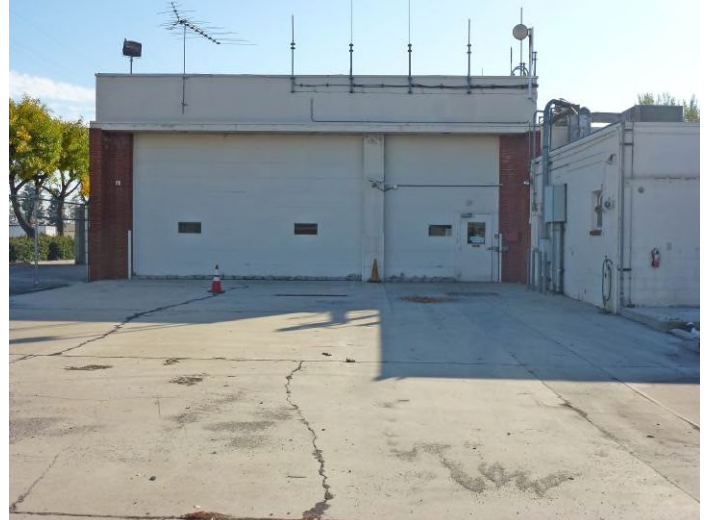
Image 6. View looking south at the north façade of the vehicle bays.
