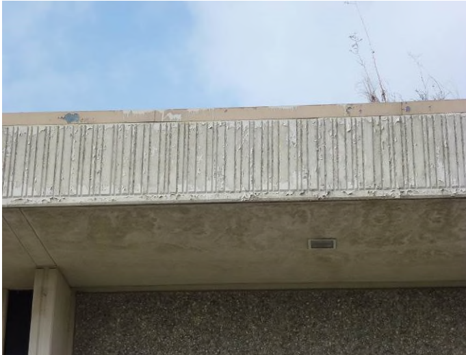
Image 5. Detail view of concrete fascia on south façade.
