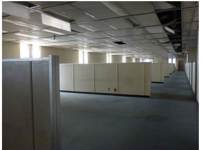
Image 8. Interior view of second floor looking southwest.
