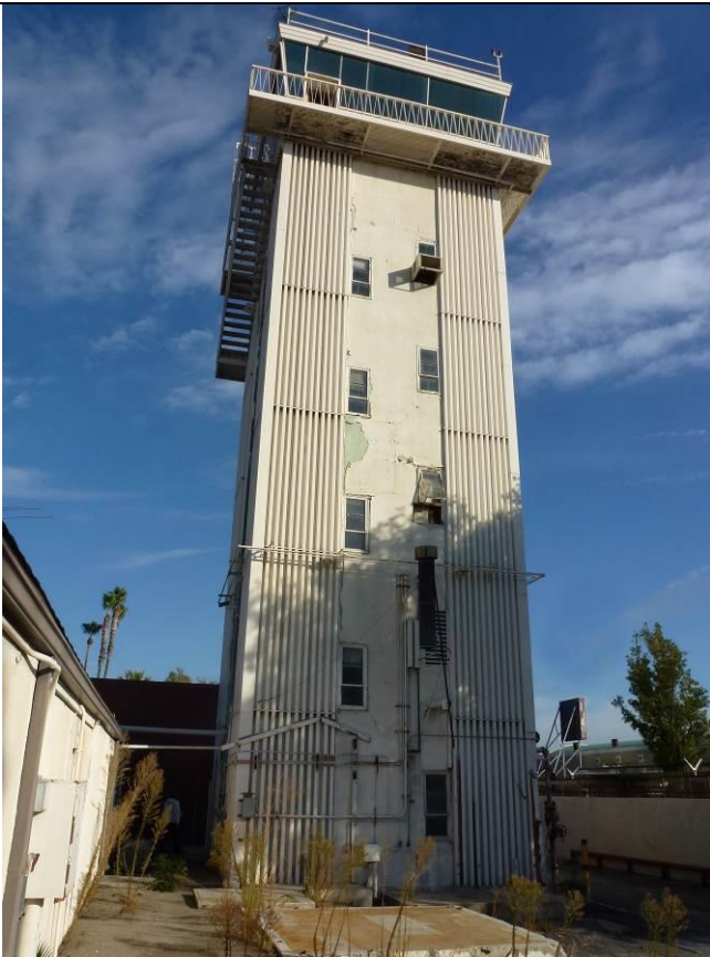
Image 3. View looking east at the west façade.
