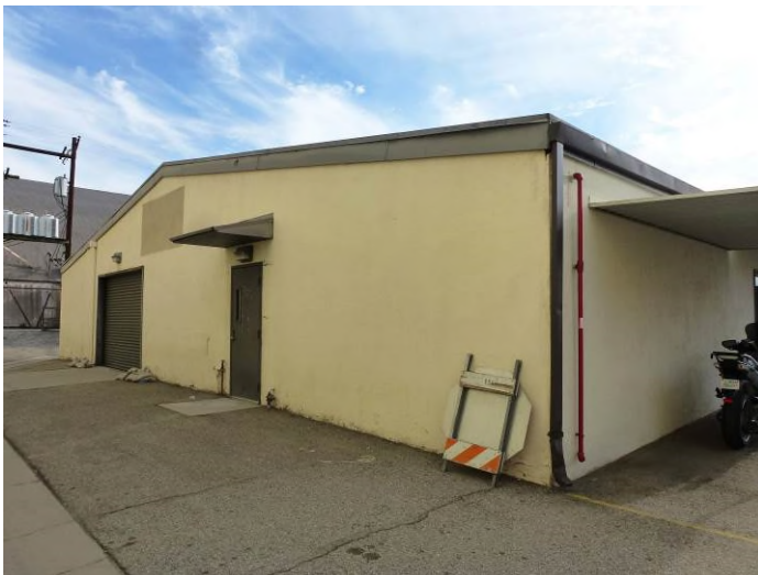
Image 1. View looking east at the northwest and southwest façades of Building E.
