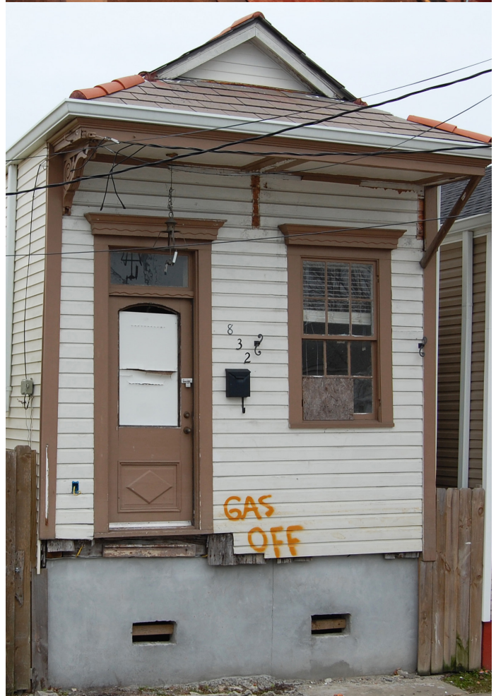
Top Left: House in New Orleans that was elevated after Hurricane Katrina.
