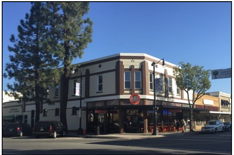
Blaze Pizza after rehabilitation, with the transoms fully restored.
