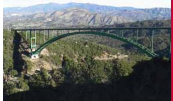
Cold Springs Canyon Bridge
