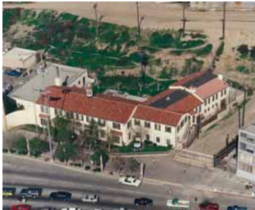
Old Custom House at the Border Southbound Pedestrian Processing and Inspection Center
